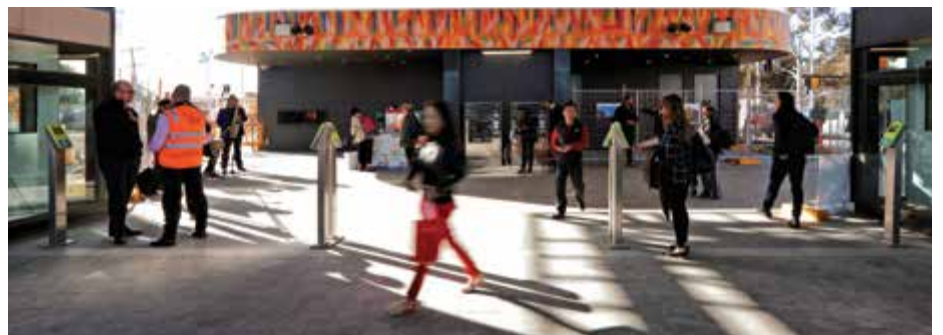
Works continue at Ginifer Station
