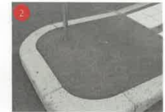
Precast concrete kerb and asphalt
