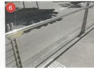
6 Yarra Trams standard barrier fencing
