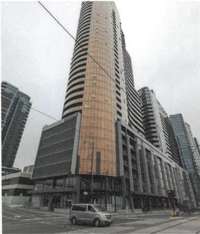
Figure 18. Example of emerging high density built form to the west (850 Whitehorse Road)
