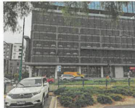
Figure 9. View from relocated tram platform to north - ATO building and multi-level car park
