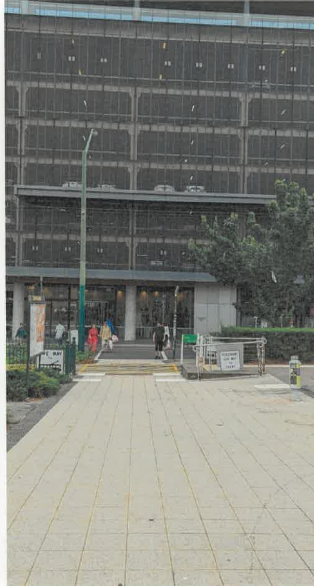
Figure 16. Pedestrian crossing within Whitehorse Road median, looking north to ATO building (Tram Terminus site located to the left).
