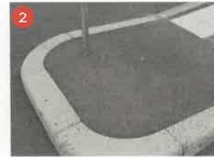
2 Precast concrete kerb and asphalt
