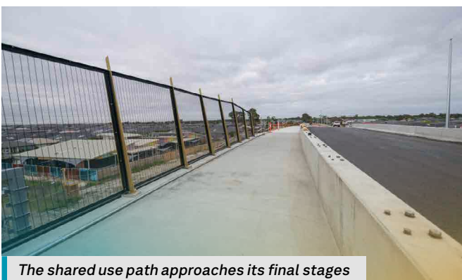
Asphalt laid over the bridge deck
