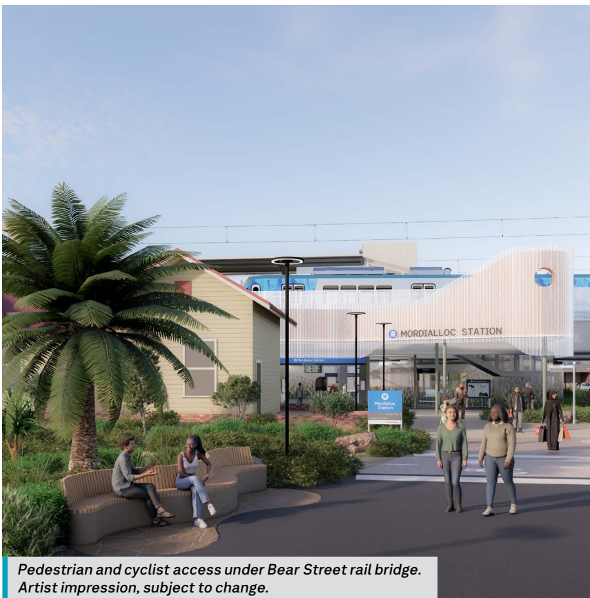
Rail bridge over McDonald Street, Mordialloc with level crossings removed. Artist impression, subject to change.
