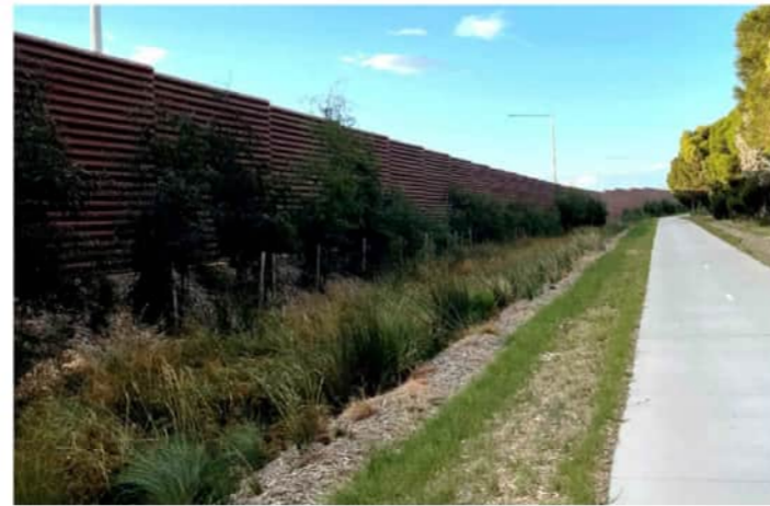
LANDSCAPE IN FRONT OF NOISE WALLS MORDIALLOC FREEWAY, BRAESIDE, VICTORIA
