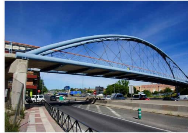
TIED-ARCH BRIDGE WITH INCLINED HANGERS
