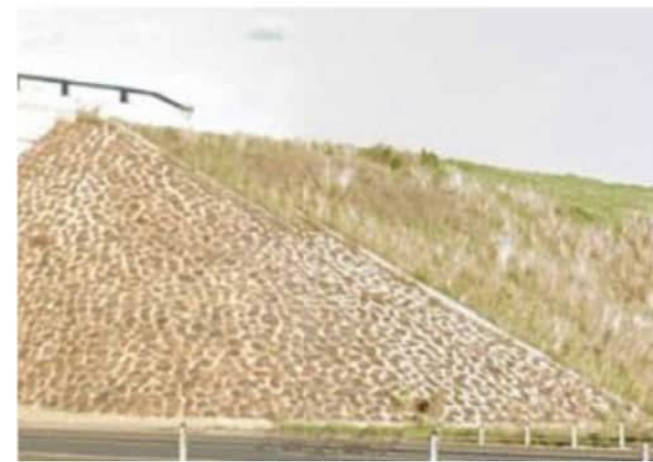
ROCK BEACHING TO REFERENCE GEOLOGY OF THE AREA
