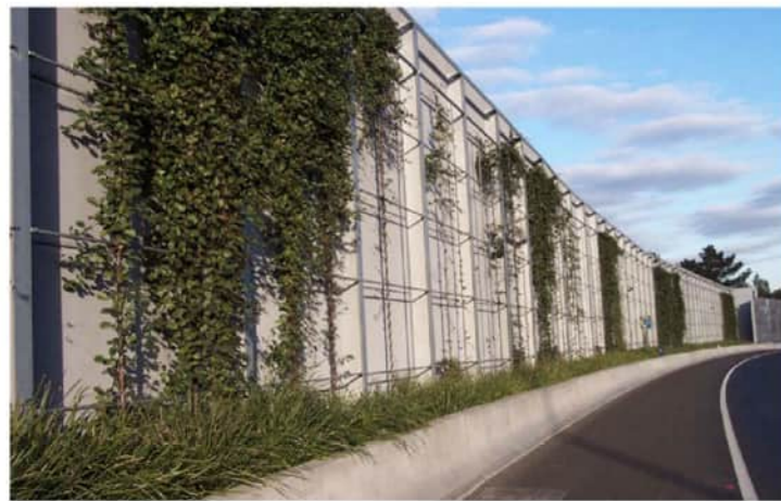
CLIMBING PLANT FRAMES SOFTEN THE VISUAL IMPACT OF NOISE WALLS IN CONFINED SPACES. TULLAMARINE FREEWAY, MOONEE PONDS, VICTORIA
