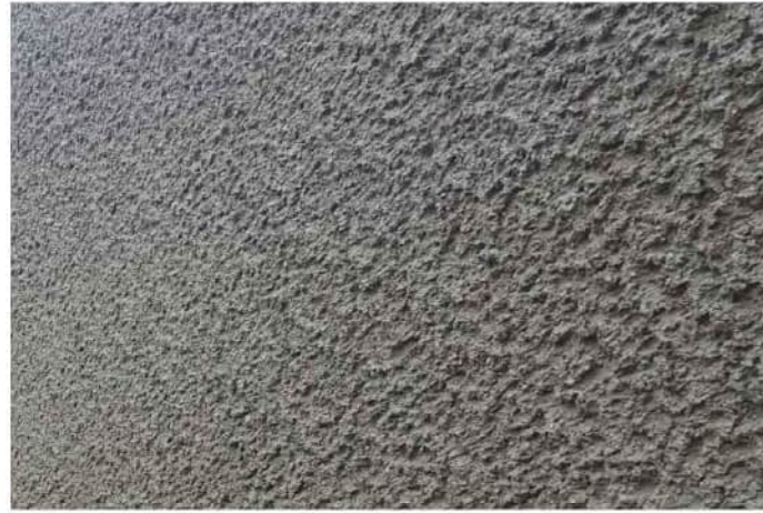
OFF-GUN SHOTCRETE FINISH
