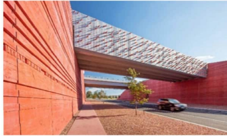
PAINT TREATMENT WESTERN HIGHWAY (REMEMBRANCE DRIVE - BALLARAT) VICTORIA
