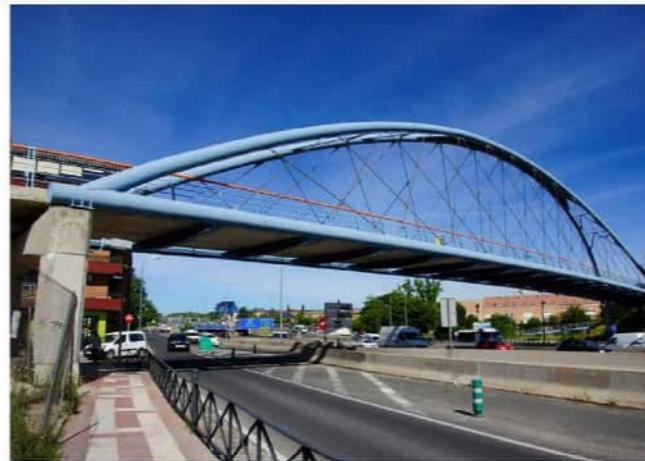
TIED-ARCH BRIDGE WITH INCLINED HANGERS
