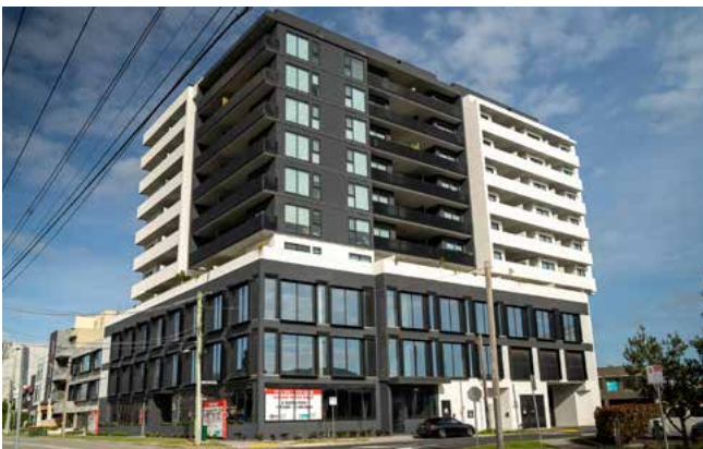
Recent office and residential development at the corner of Jamieson Street and Chesterville Road, Cheltenham
