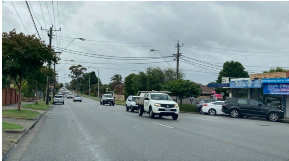
Small, fine-grain commercial buildings built to the boundary (0 to 1 metre setback) on Chesterville Road
