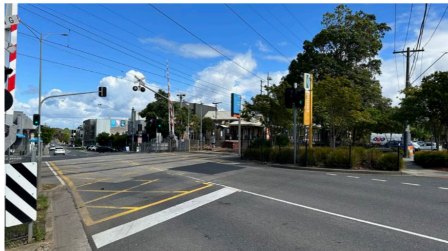
Level crossing at Highett Station
