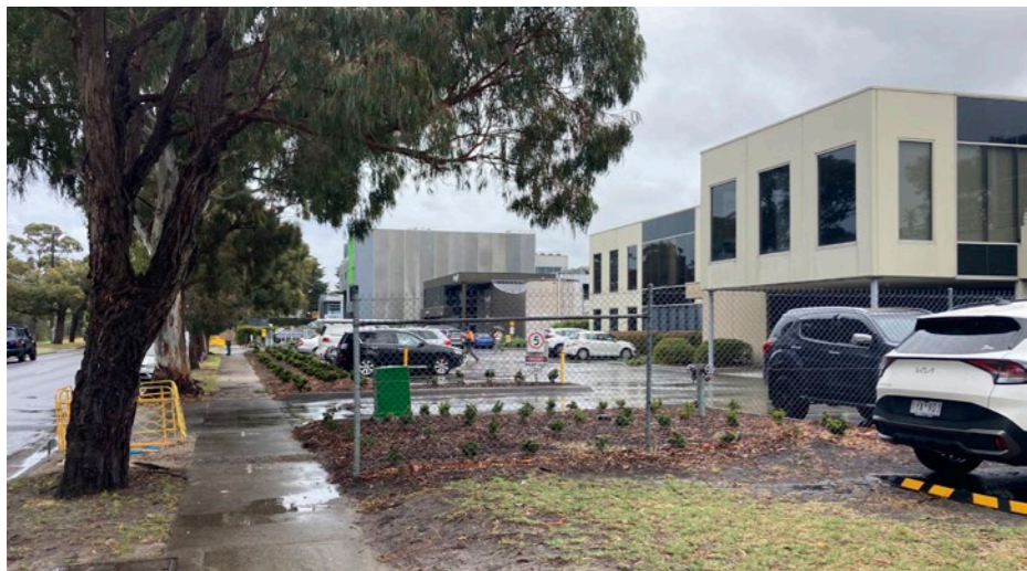
Large format commercial and industrial buildings with setbacks >15 metres located within Bayside Industrial Area
