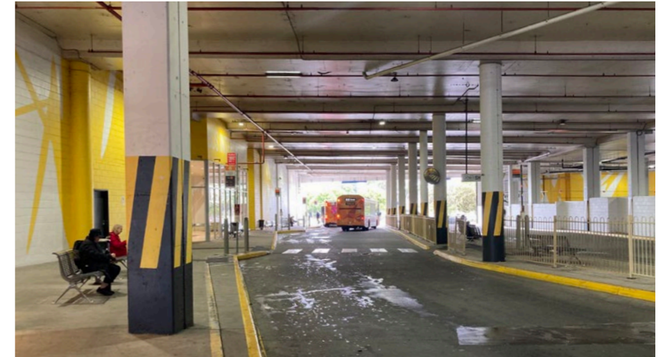
Southland Shopping Centre bus interchange
