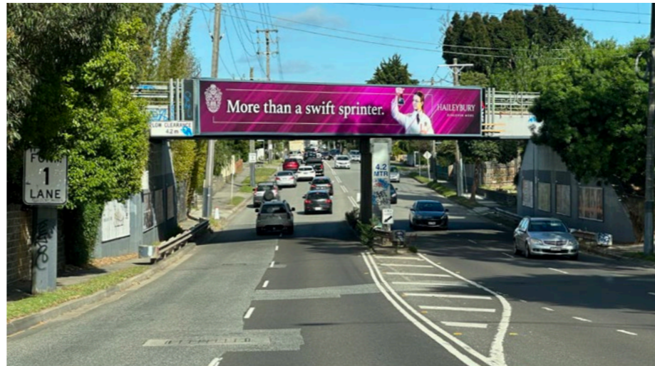
Bay Road pedestrian / vehicle underpass
