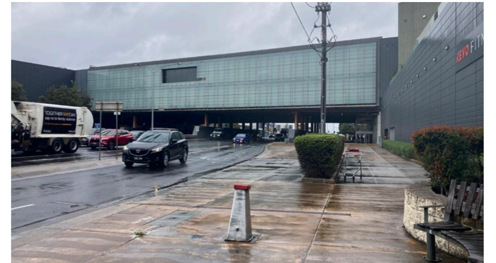
Southland Shopping Centre pedestrian experience at Nepean Highway
