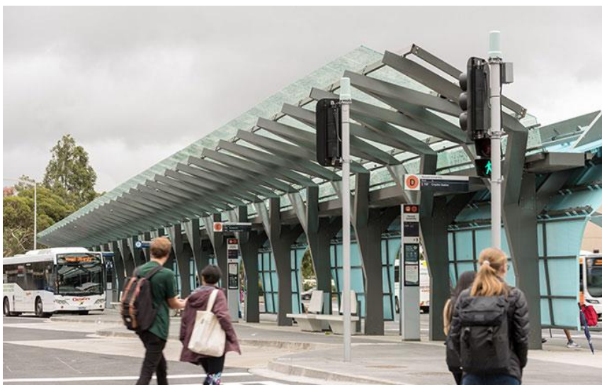
FIGURE 2.16 MONASH UNIVERSITY BUS INTERCHANGE (SOURCE: MONASH UNIVERSITY)
