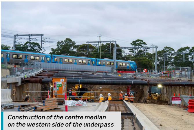
Excavation between temporary steel braces, used to support the walls of the underpass
