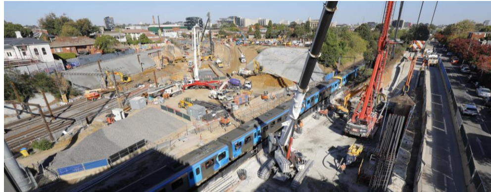
Piling at Osborne Street
