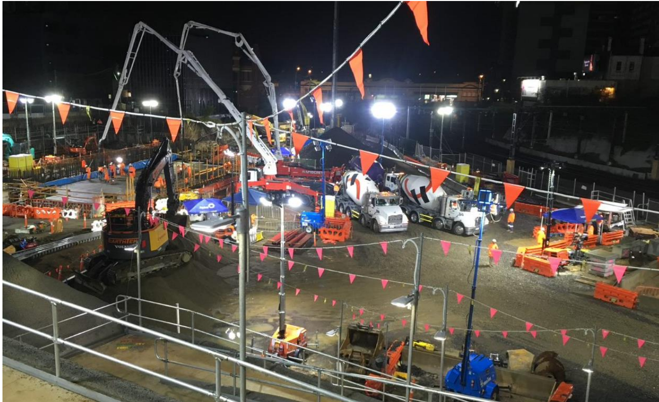
Pouring the concrete for the roof slab
