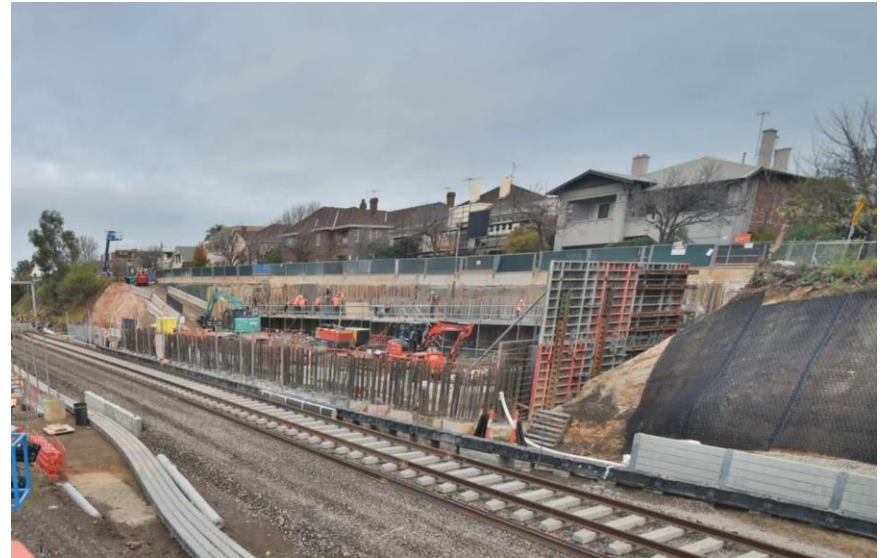
Construction of the TBM retrieval shaft
