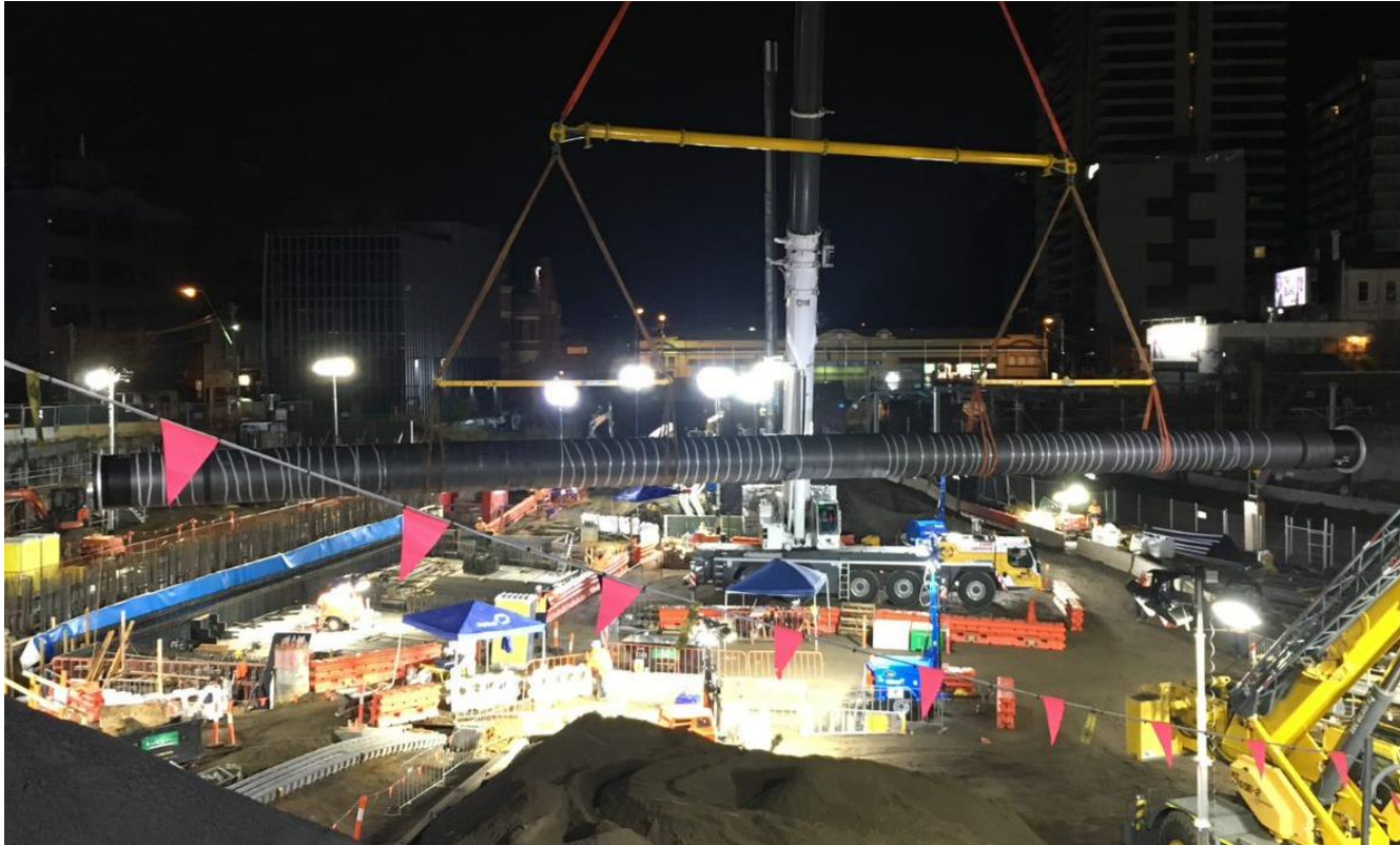
Installing the drain pipe
