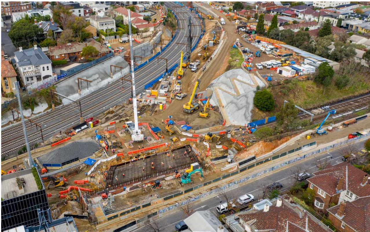
Preparing the roof slab
