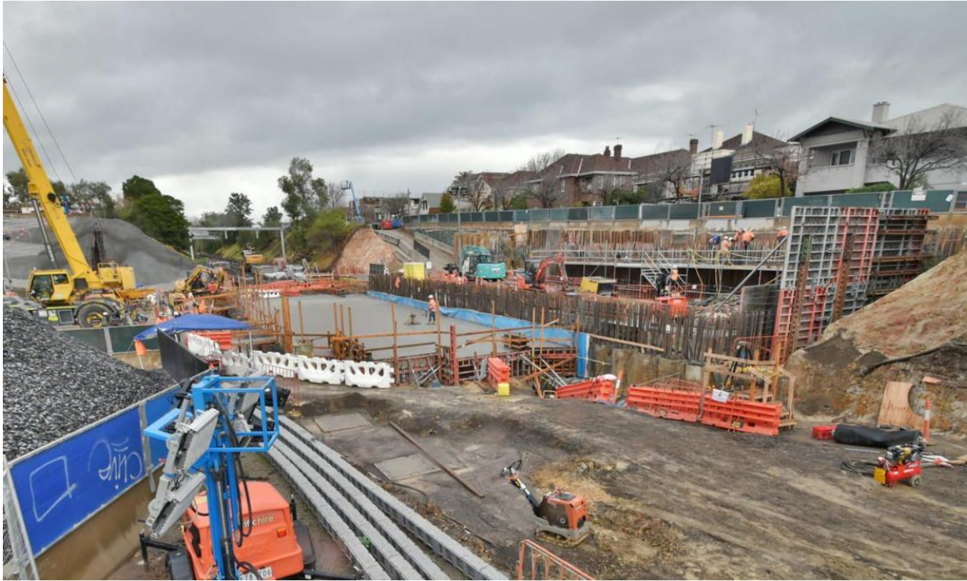
The tunnel roof slab
