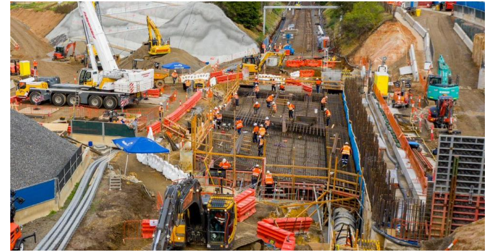
Preparing the roof slab
