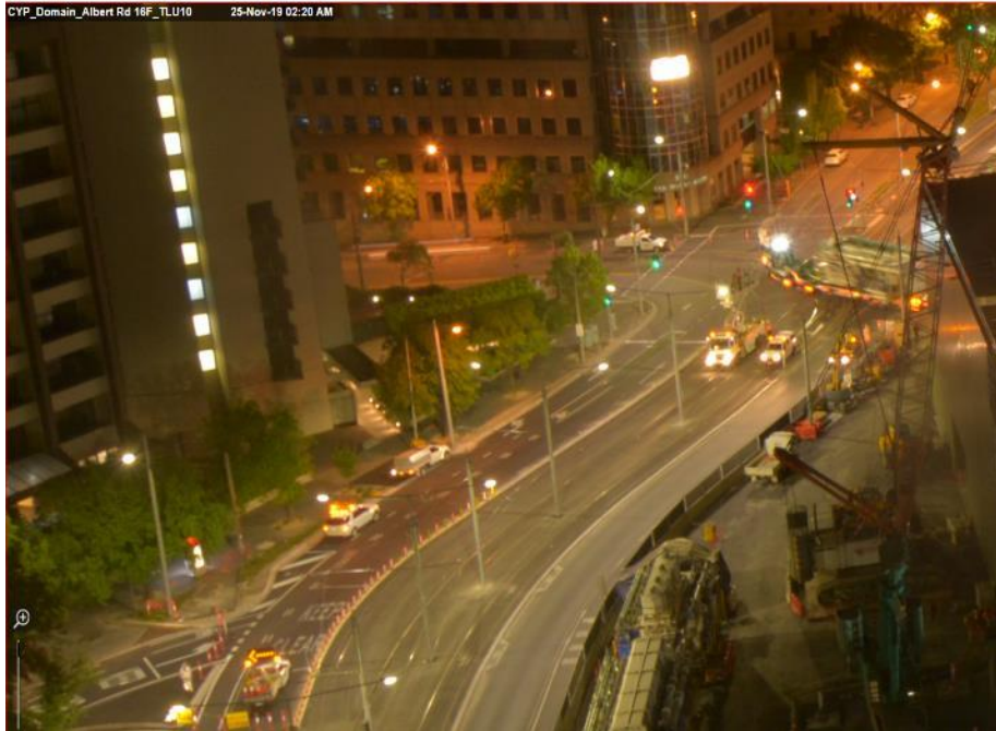
TBM Delivery 25/11 – 2:20am
