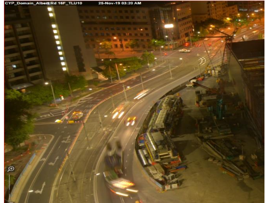
TBM Delivery 25/11 – 3:20am
