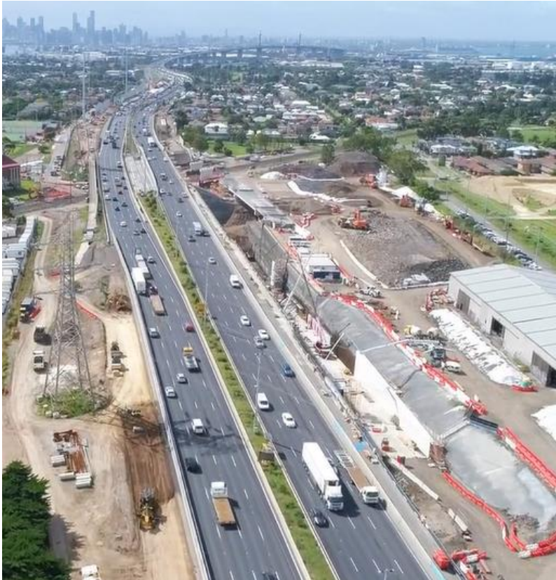
Newport Rail Bridge and Southern outbound Portal construction works
