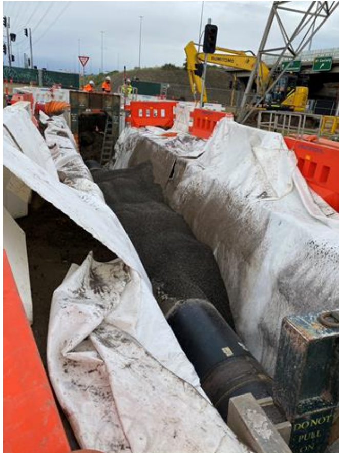
Utility works inbound exit ramp
