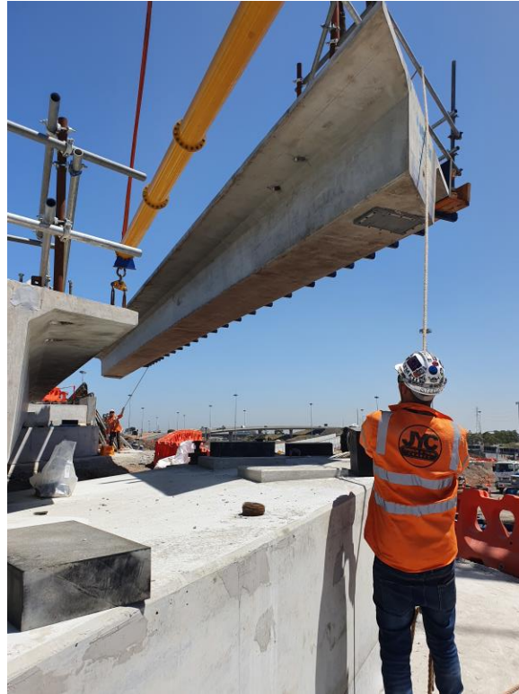
Deck barrier installation
