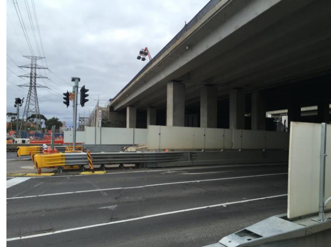
New northern piers and bridge structures
