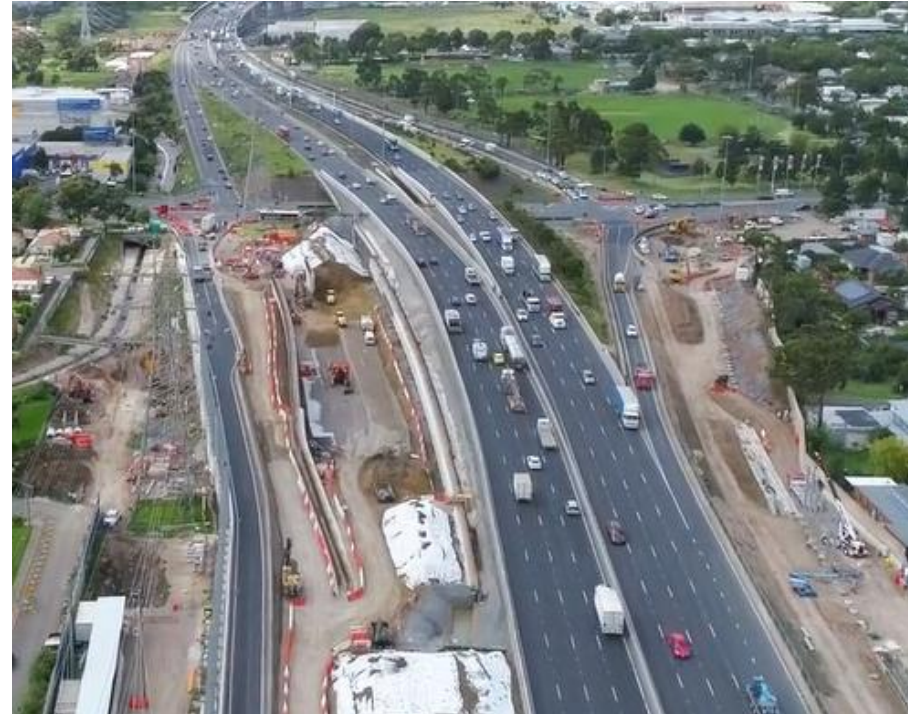
Williamstown Road and Northern inbound Portal construction works
