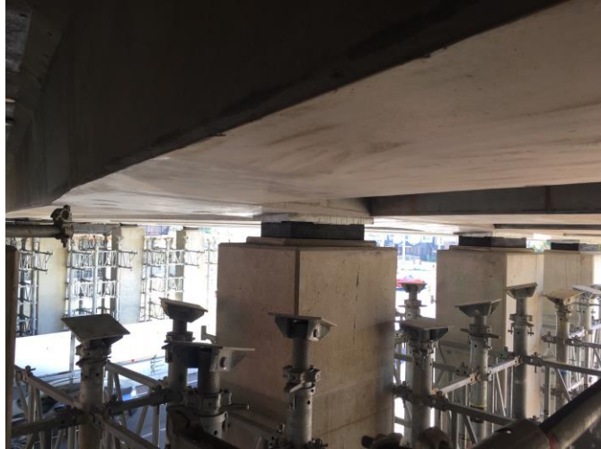
New piers and abutment bearing replacement
