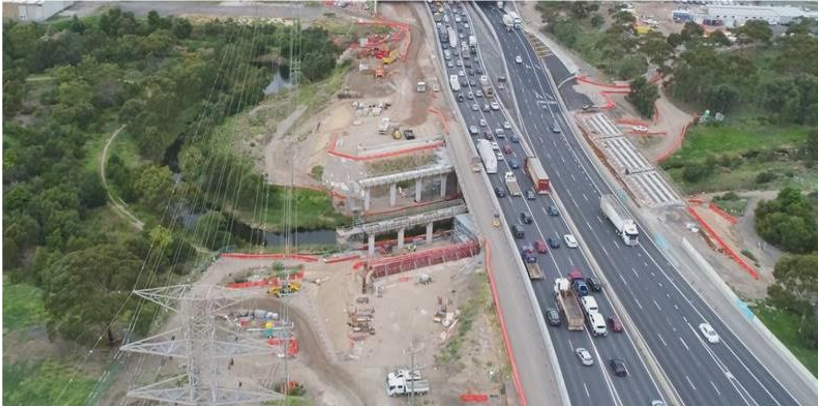
Kororoit Creek Bridge strengthening and widening works
