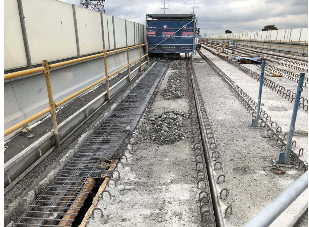
Acoustic panels surround the mobile scaffold which houses the hydro-blasting robot
