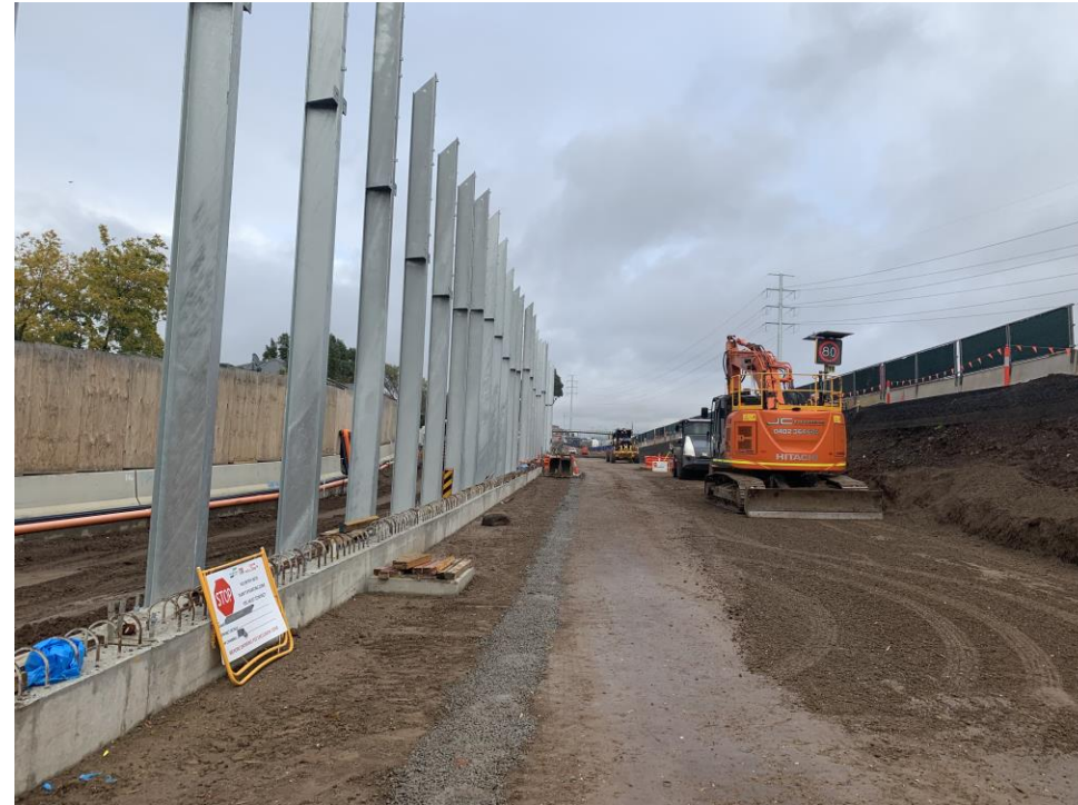
Pavement preparation works on the outbound entry ramp
