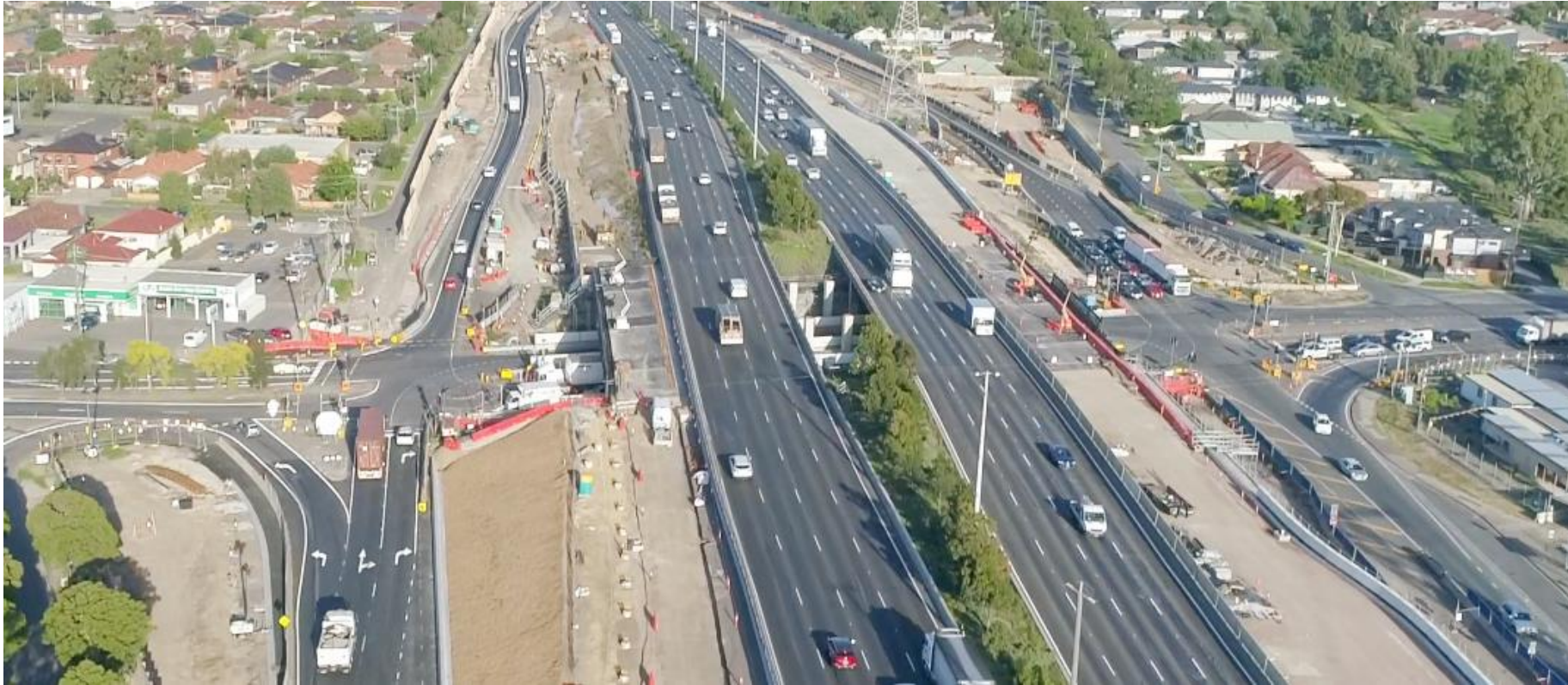
Freeway widening works at Millers Road Interchange
