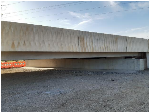
Top down bridge pre excavation
