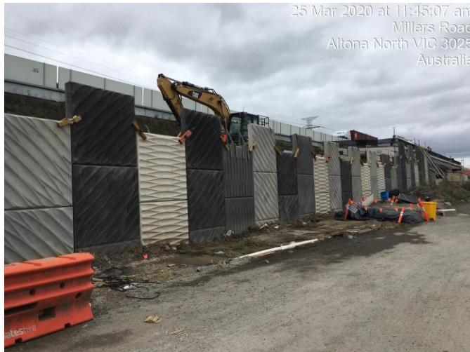
Reinforced Soil Structure retaining wall under construction
