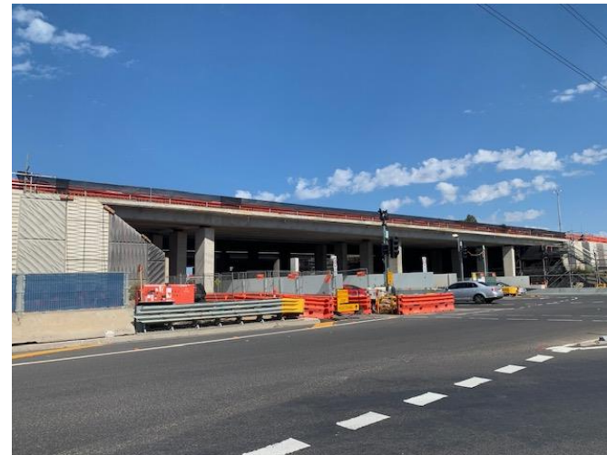
New northern piers and bridge structures
