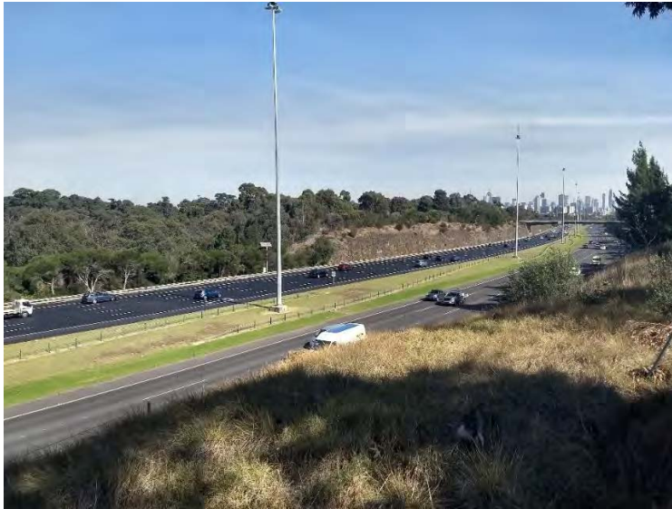
Figure 6-15 Open landscape character of the Eastern Freeway within Precinct 3.F
