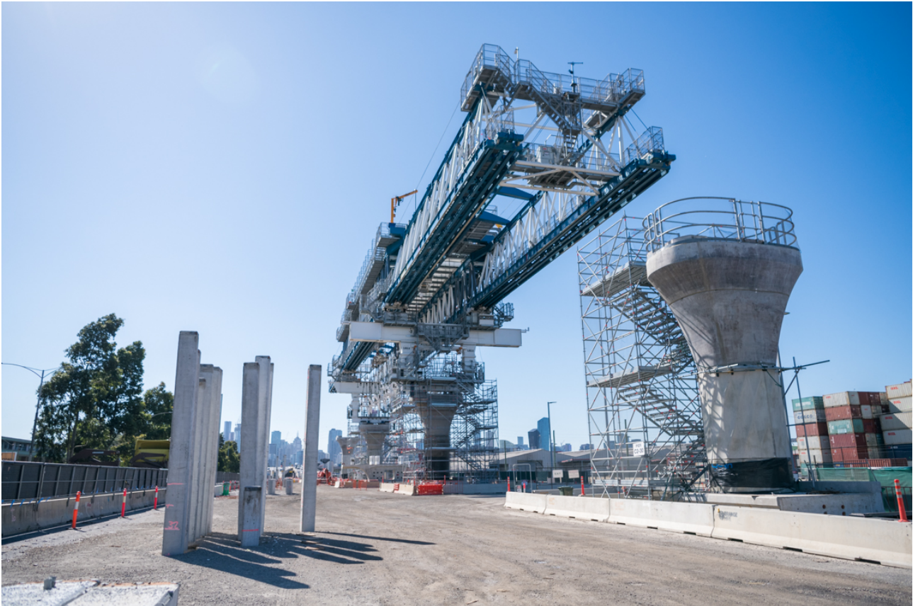
Photo 1 – Launching gantry and precast column works along Footscray Road – East Zone (Source: WGTP MTIA, 18 February 2021)
