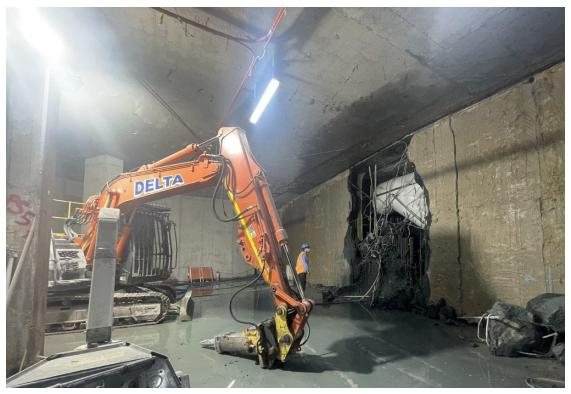
D-wall demolition between station box and Shrine of Remembrance station entrance
