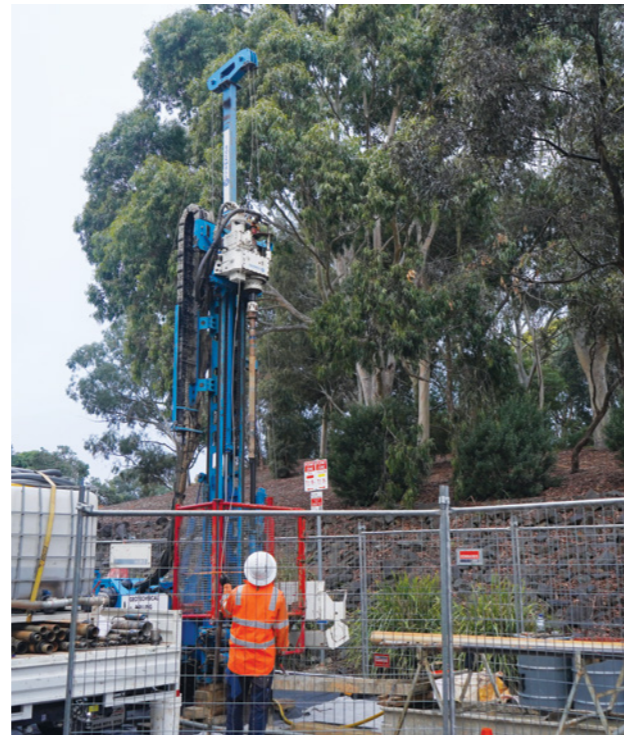
SRL East site investigations at Monash University
