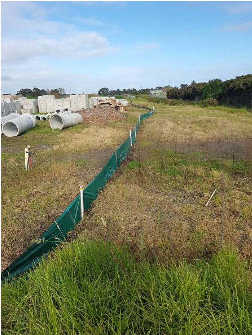
Left: The sediment fence south of Zone 1, Gate 4 was extended, as required by the previous audit recommendation.
