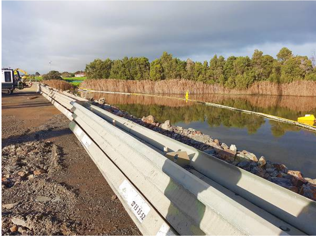
Above: Silt curtains around the Waterways piling platform appeared effective in containing sediment.
