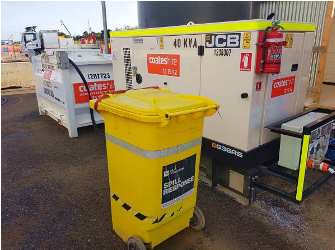
Above: Compliant example of spill kits located next to generator at waterways compound Below: Complaint example of labelled bins at waterways compound.
