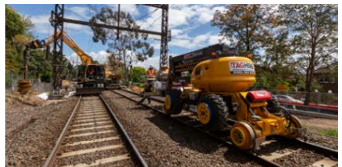
Installing new overhead wiring structures
