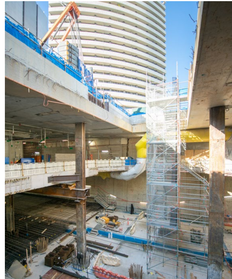
Base slab construction, concourse level and roof slab of station box
