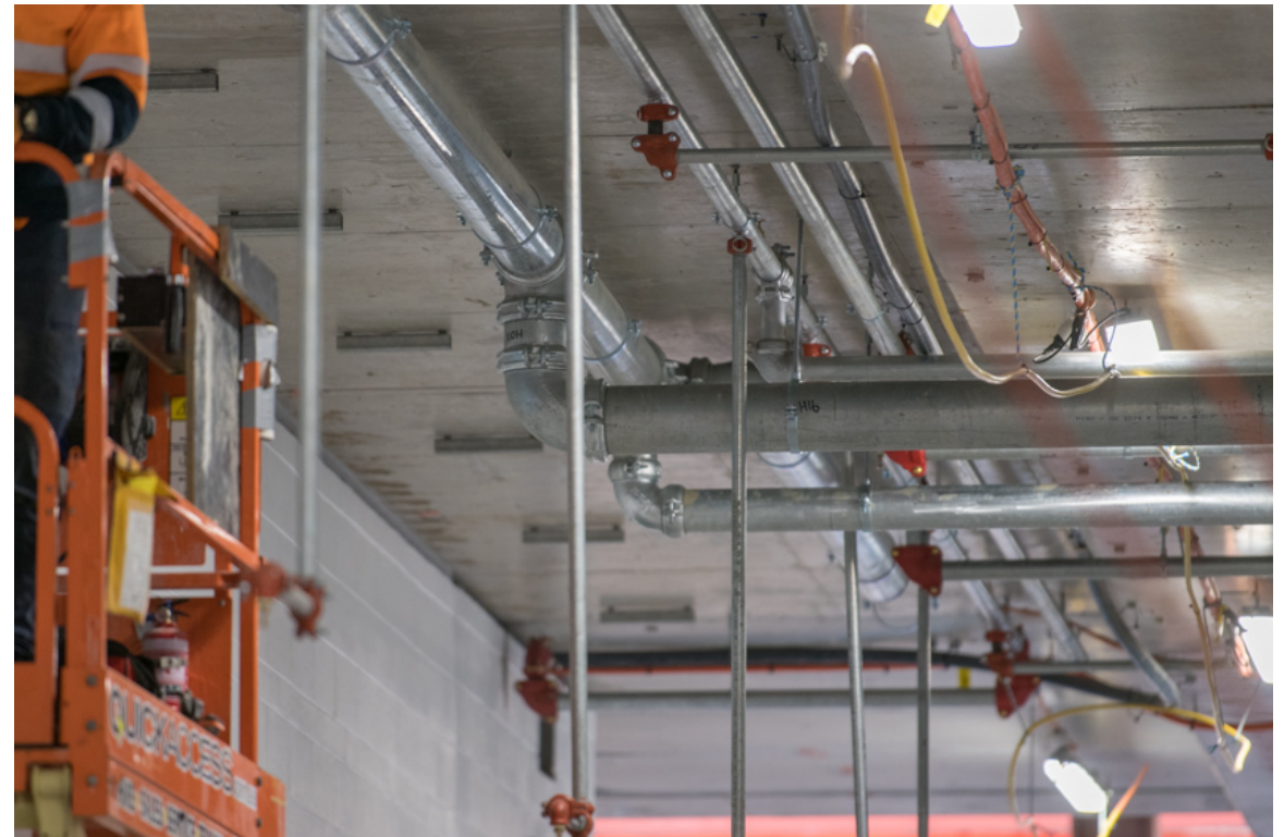
Mechanical, electrical and plumbing rough-in – service building
