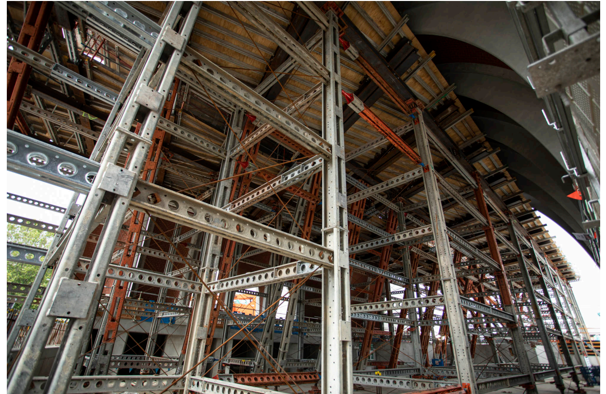
Support structure for arches being removed
