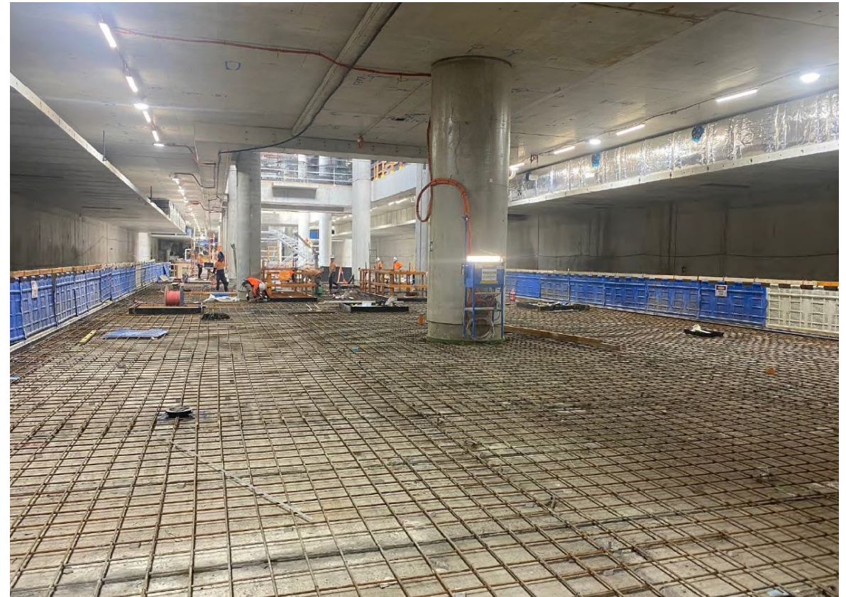
Platform topping slab construction
