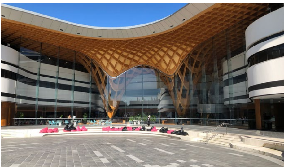
Reference 1. Bunjil Place, Narre Warren VIC The built form of the community centre evokes Bunjil the Creator of the Kulin Nation
