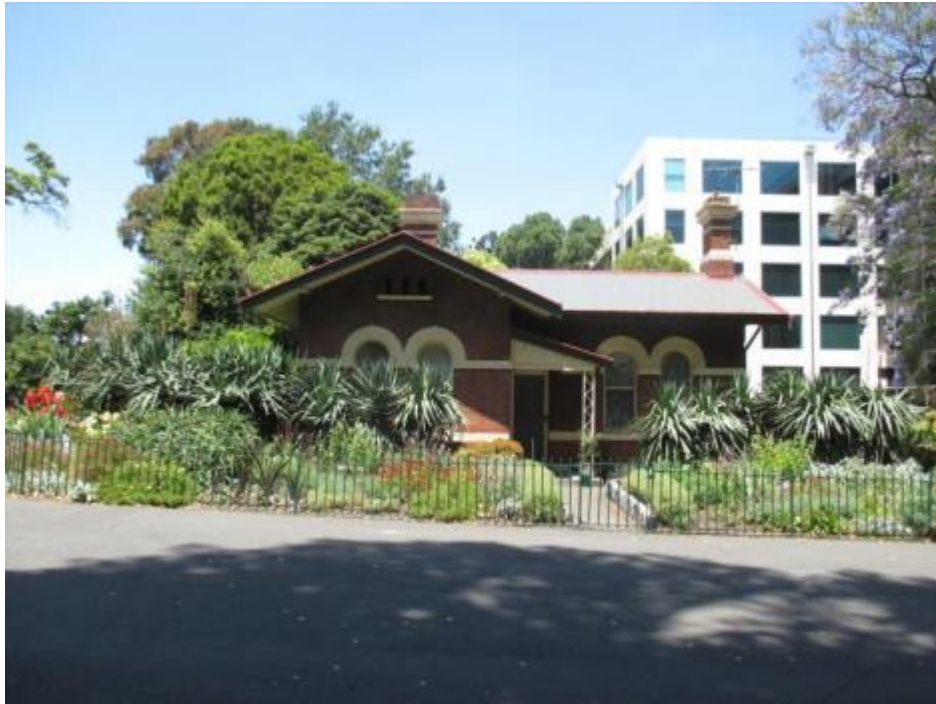
Caretaker's Cottage on the western edge of Fawcner Park as viewed from the north; note the low iron fence and cottage-style garden
