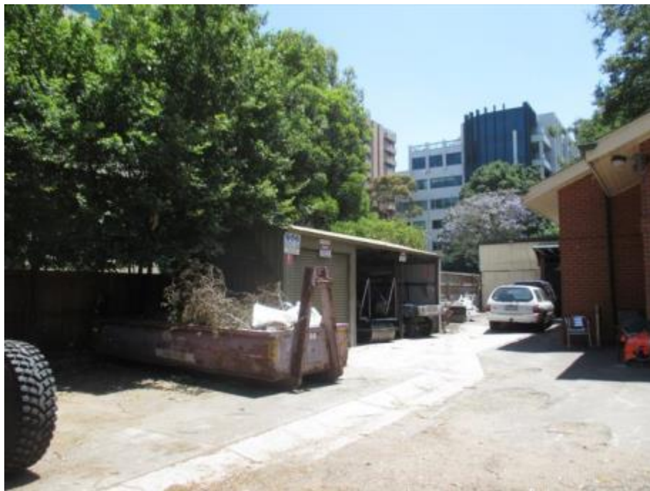
Sheds and lunchroom structure in the works depot to the south of the Caretaker's Cottage
