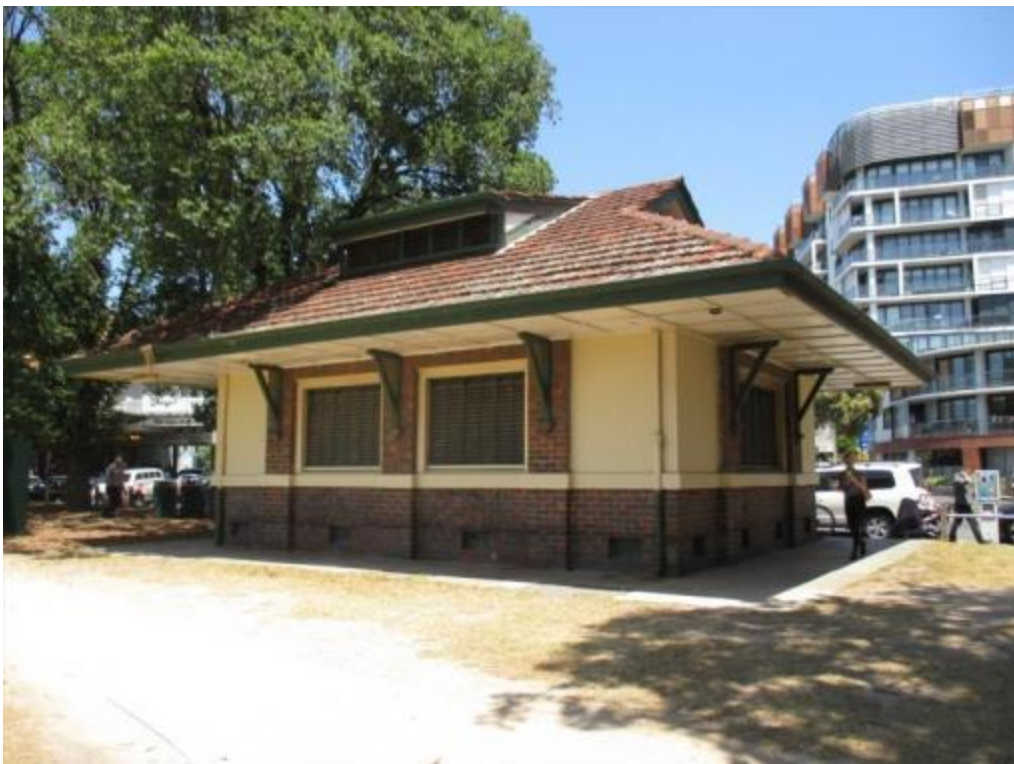
Substation at the southern edge of Fawkner Park, as viewed from the north-west
