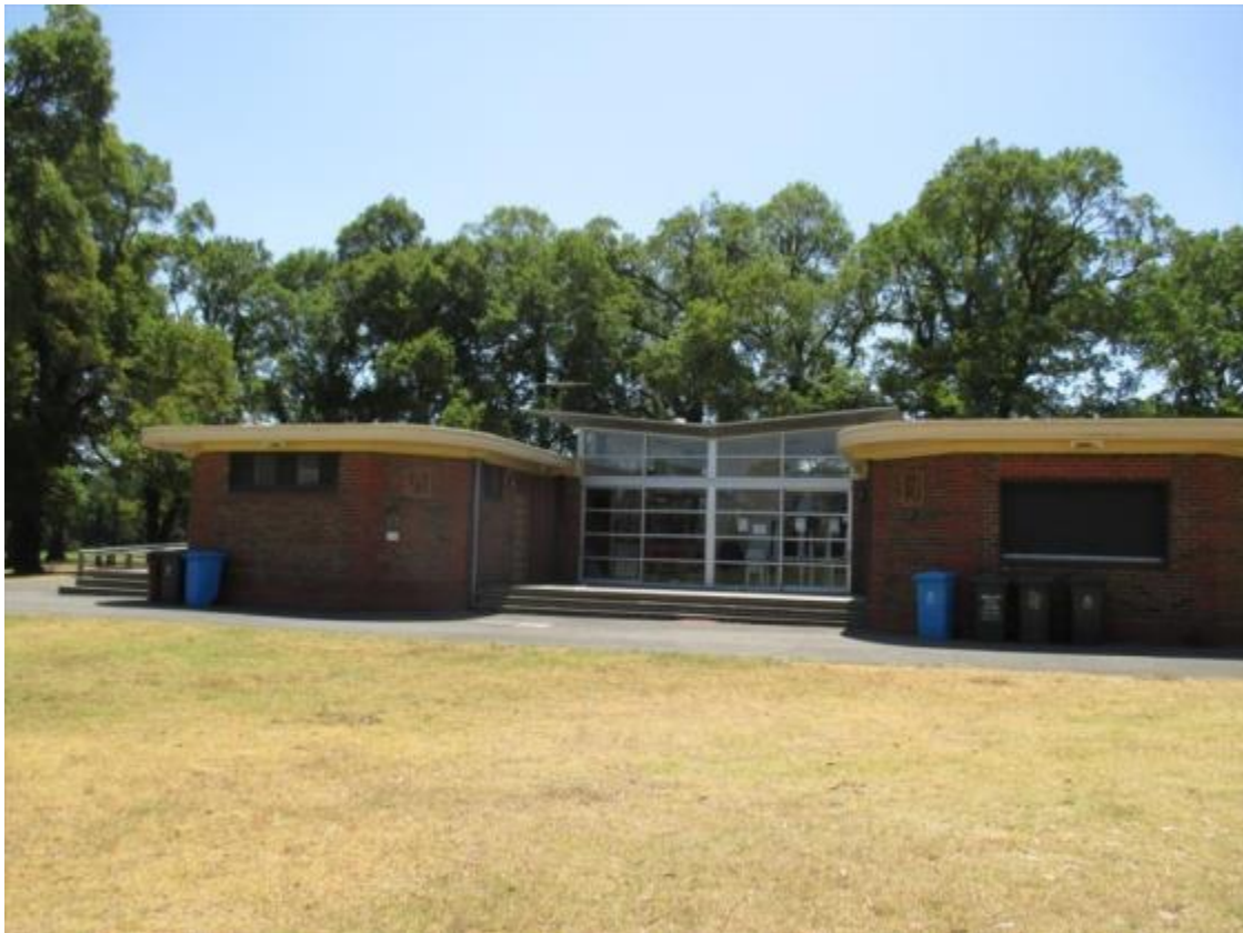
Northern pavilion, showing recent butterfly roofed addition, as viewed from the south-west
