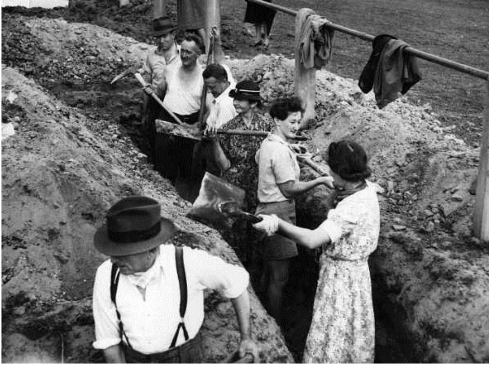
Air raid trench digging Fawkner Park South Yarra, c. 1942
