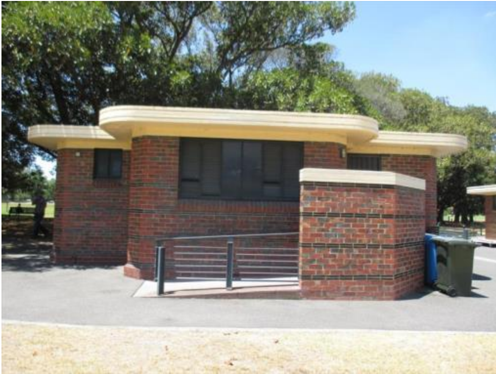
Southern toilet block (now store) viewed from the west
