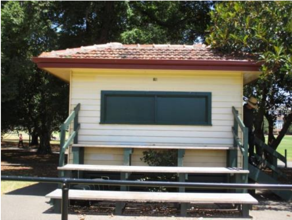
Timber scoreboard building located to the south-west edge of Cordner oval
