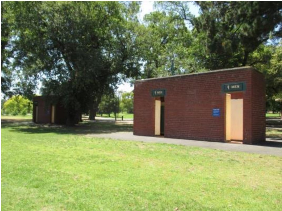
Northern toilet blocks (interwar), viewed from the lawns to the west
