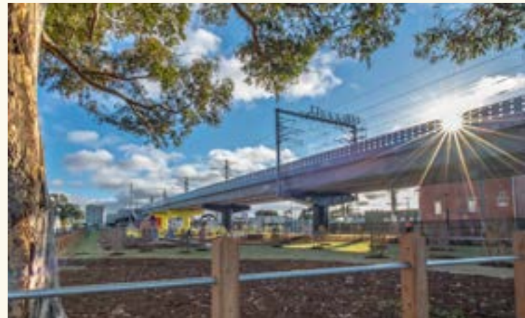
Moreland open space and elevated rail
