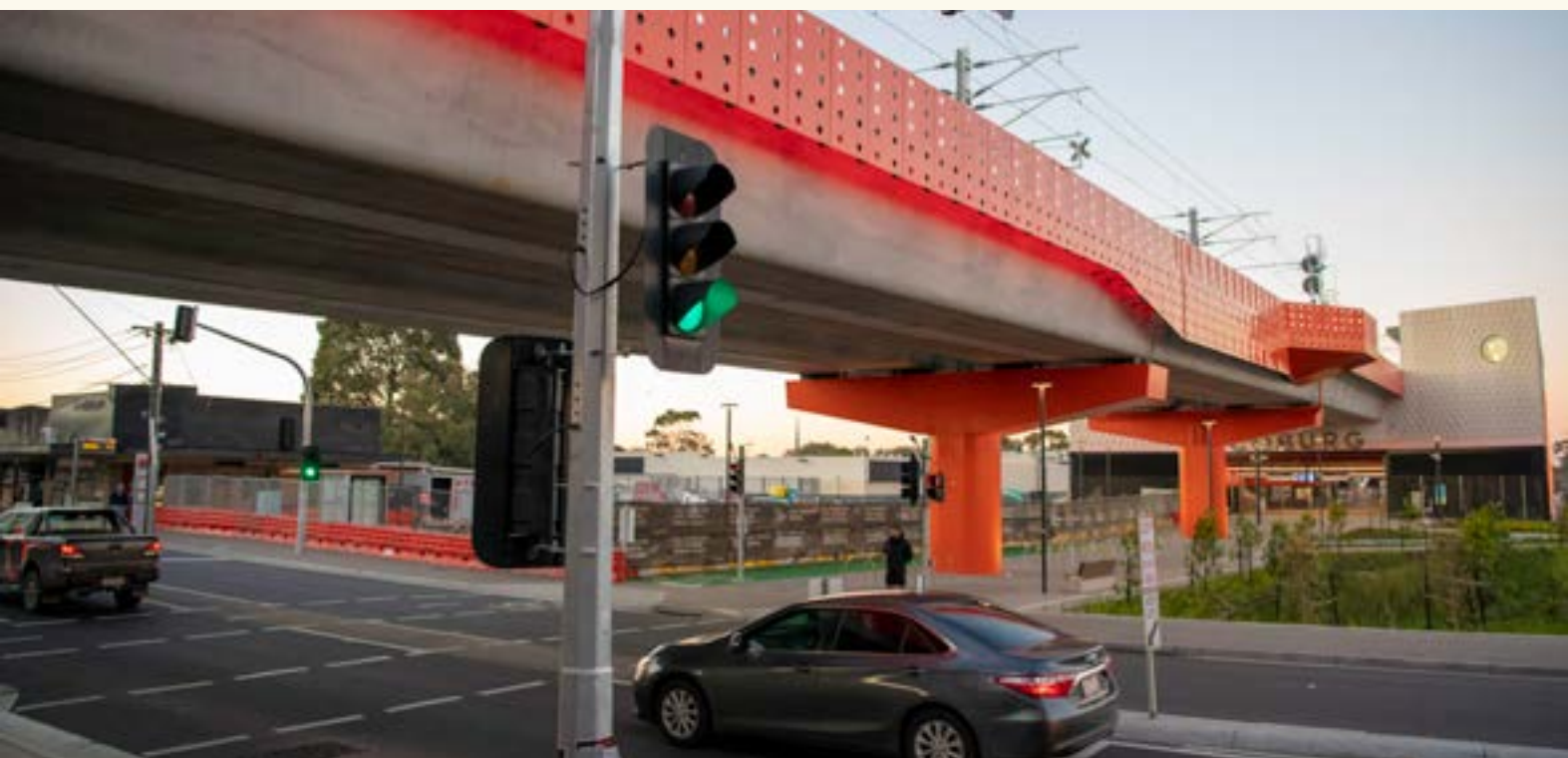
New rail bridge over Bell Street, Coburg
