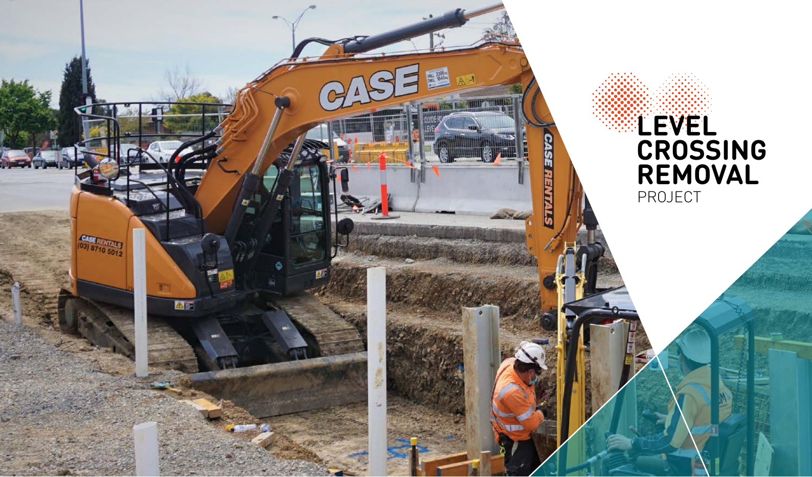
Excavation works in preparation for the new road underpass
