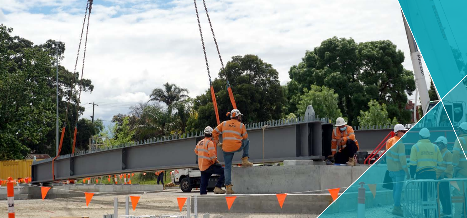
The steel bridge beams being delivered to site
