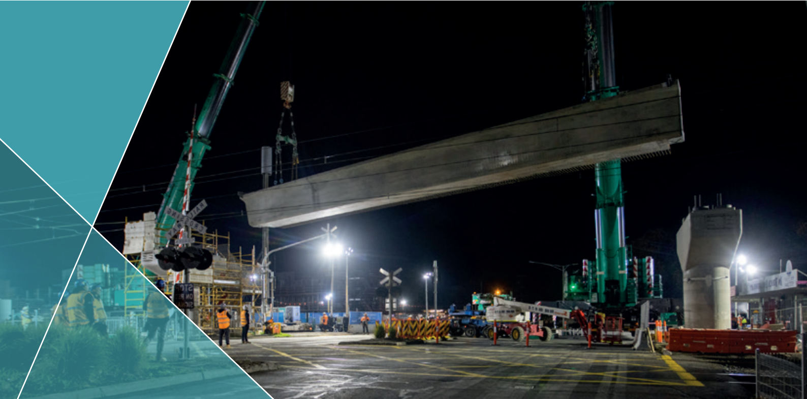
L-beam installation at Manchester Road, Mooroolbark
