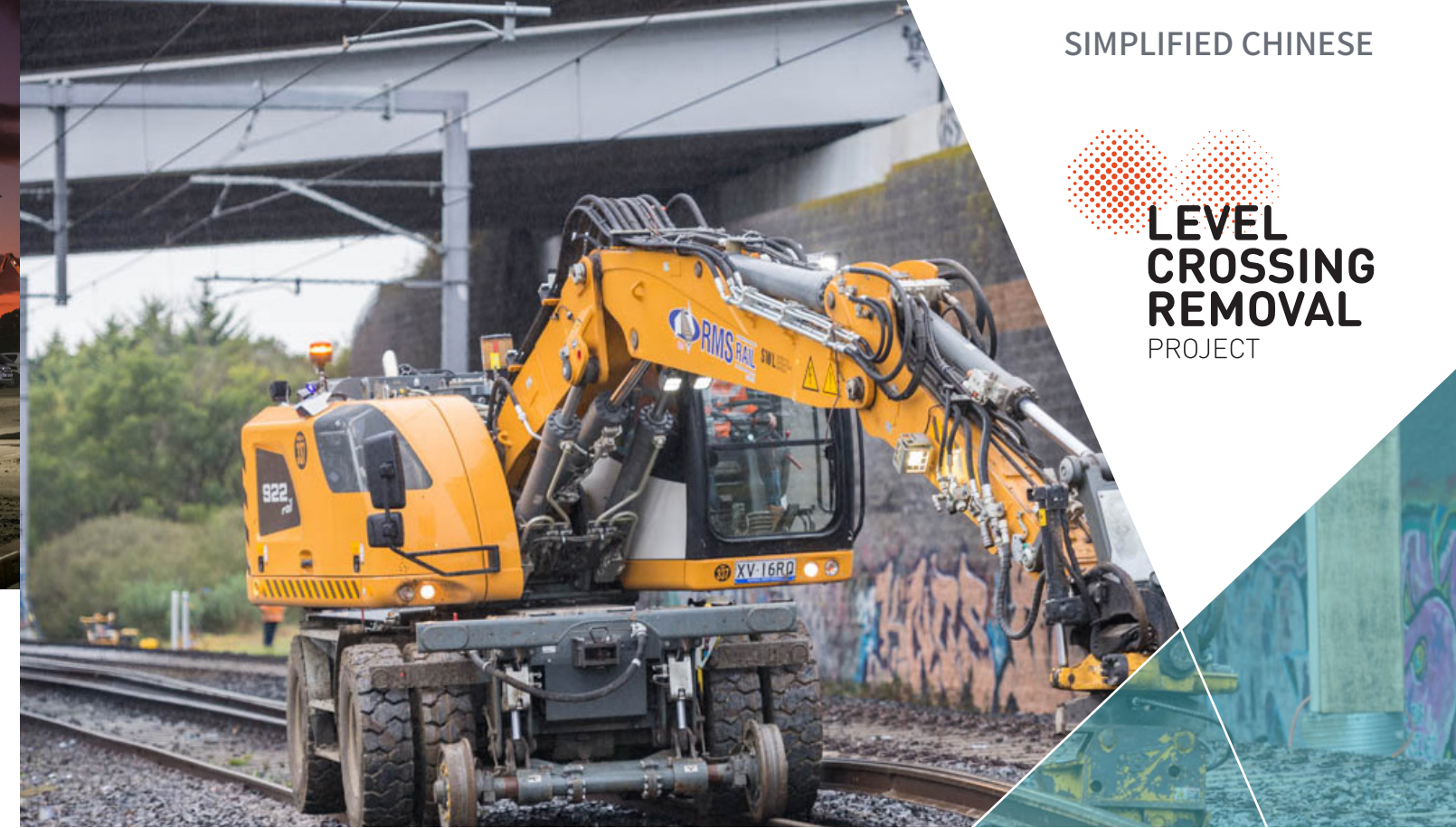
专用挖掘子在East Pakenham为拖曳铁轨做准备
