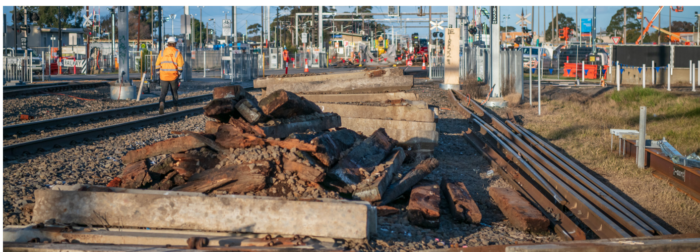
拆除Main Street平交路口的铁轨和枕木
