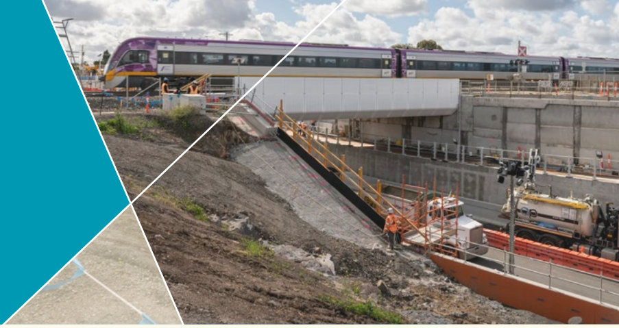
Finishing touches on the new Robyns Road underpass
