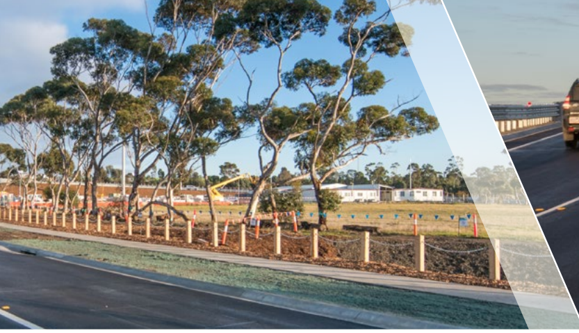
New Fitzgerald Road bridge
