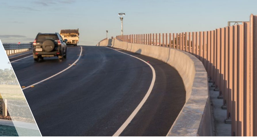
First cars over the new Fitzgerald Road bridge
