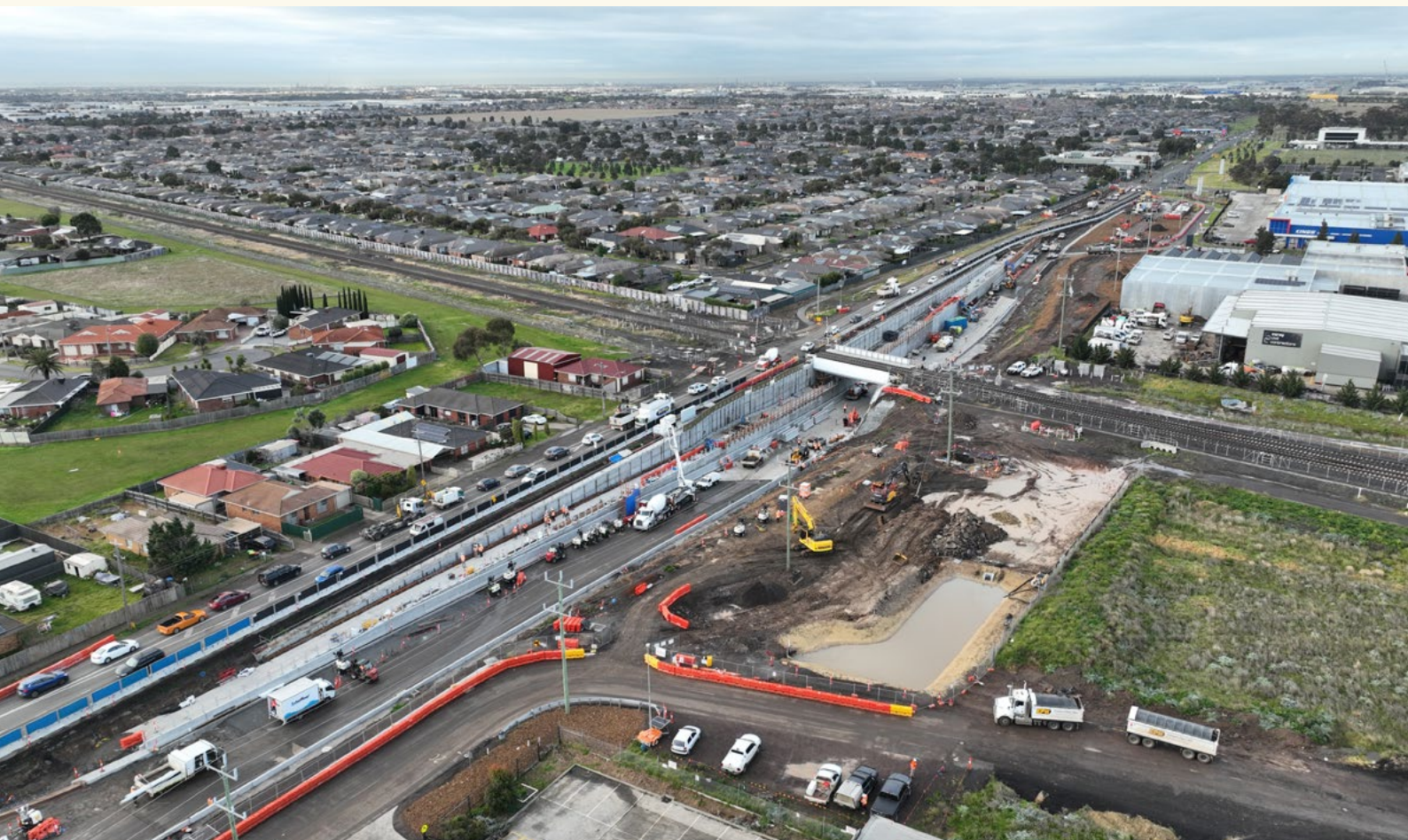
Aerial view of Robyns Road during major works
