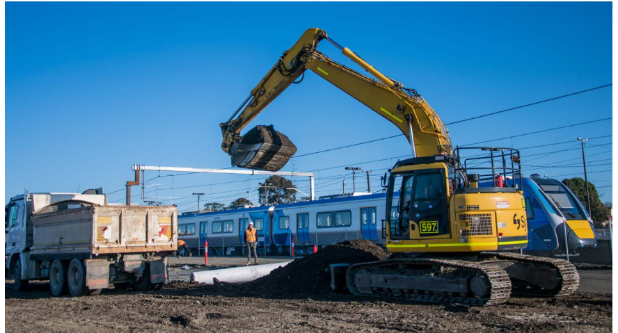
Excavating and hardstand construction works at Pakenham Station.
