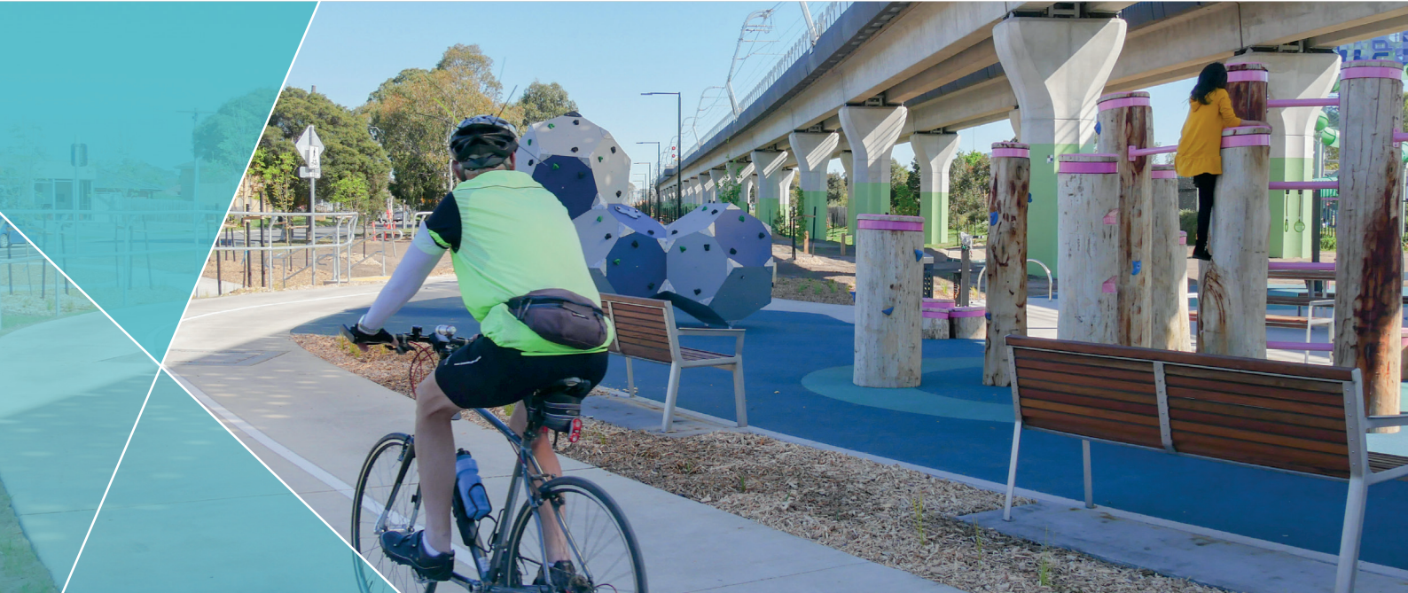
A cyclist using the shared path built as part of the Caulfield to Dandenong project.
