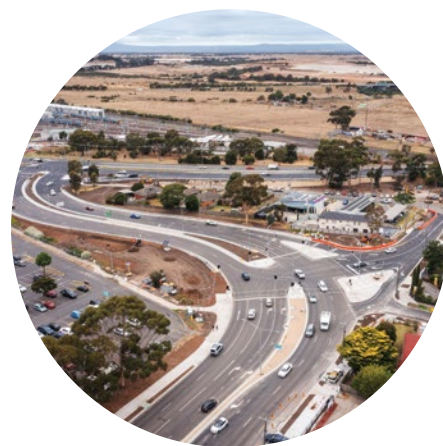
Image: Newly completed Craigieburn Road to the Hume Highway
