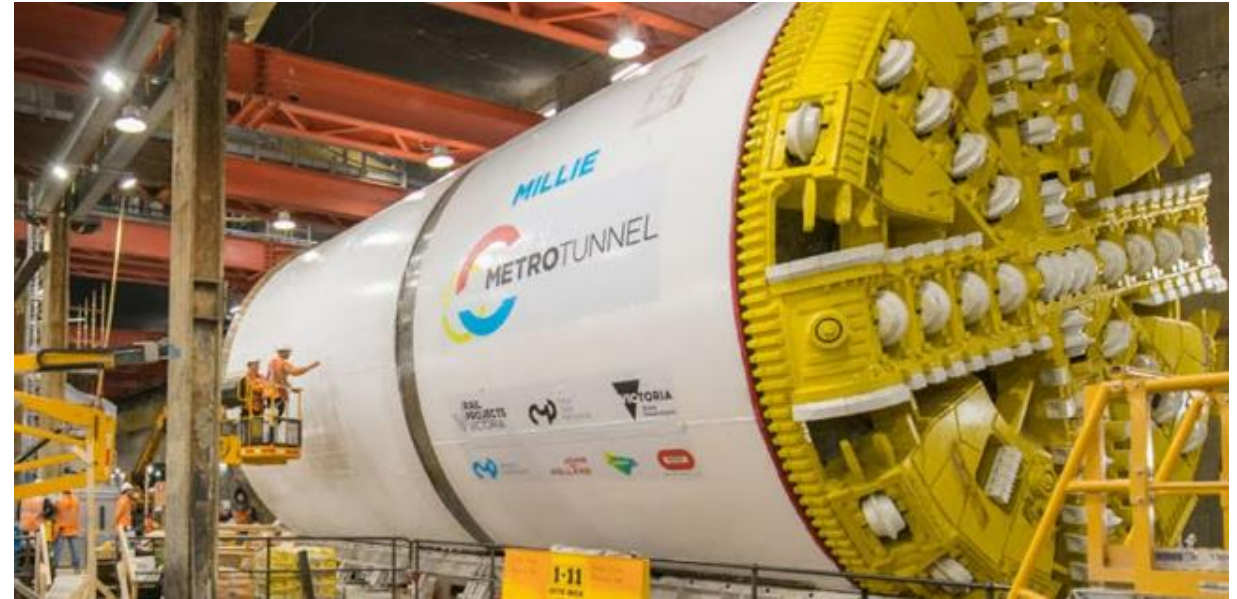
Image: Metro Tunnel Project Tunnel boring machine
