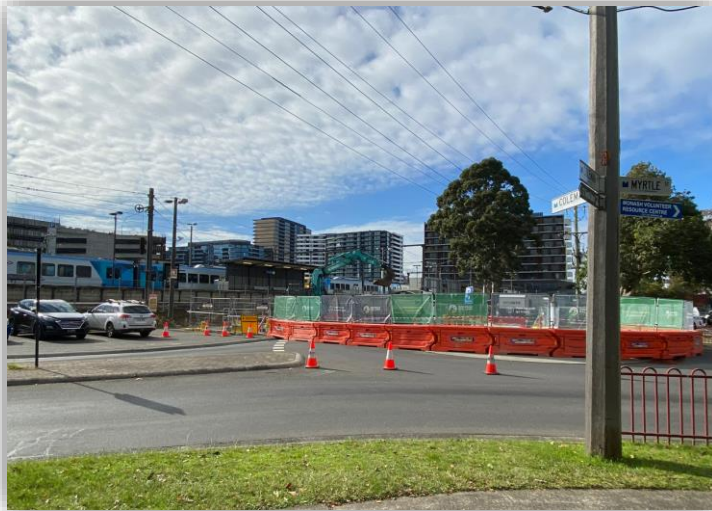
Water relocation in Glen Waverley
