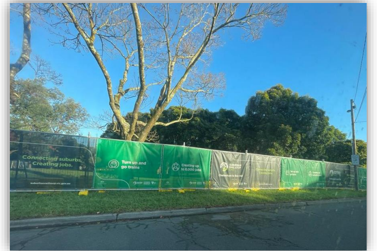
Site establishment in Burwood
