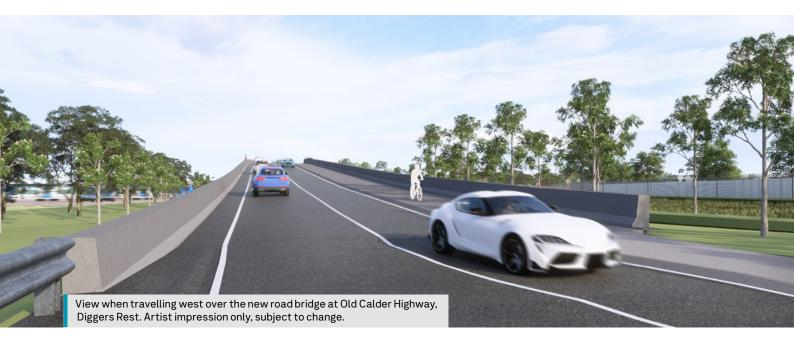
At Old Calder Highway, the new road bridge will start south of the existing level crossing and connect Old Calder Highway to Diggers Rest-Coimadai Road.
