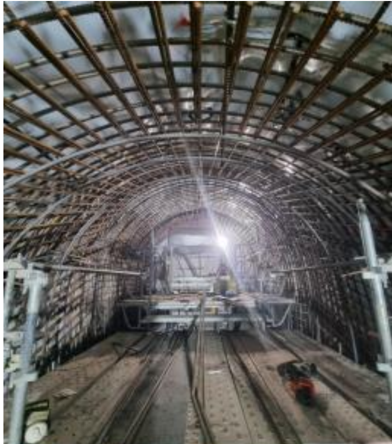
Cross Passage Three – Reinforcements
