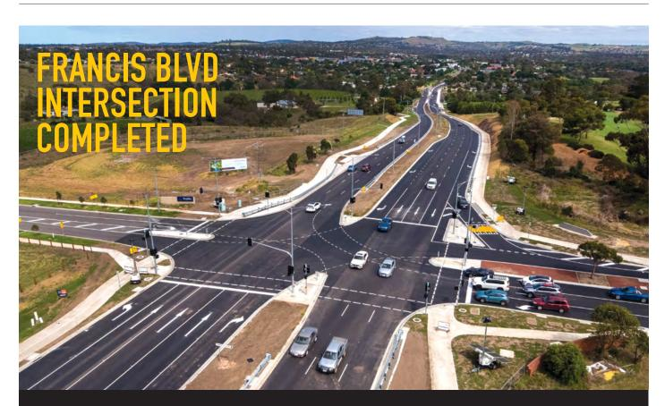
We've installed new traffic lights to replace the roundabout at Francis Boulevard. This will allow more vehicles to travel through the intersection during peak times and provide more reliable journeys. A new pedestrian crossing links new walking and cycling paths and will provide easier access for walkers and cyclists.
