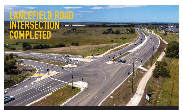
The widened and upgraded intersection can better accommodate the large number of heavy vehicles using this intersection. Traffic lights improve safety for all motorists travelling along Sunbury Road, and provide a safe location for U-turns.
