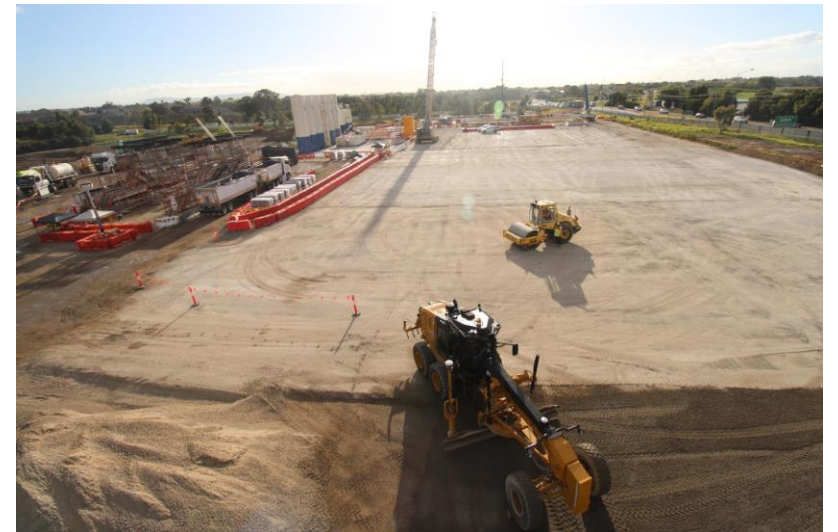
Image above: Bentonite plant and piling rigs at 217 Kingston Road
