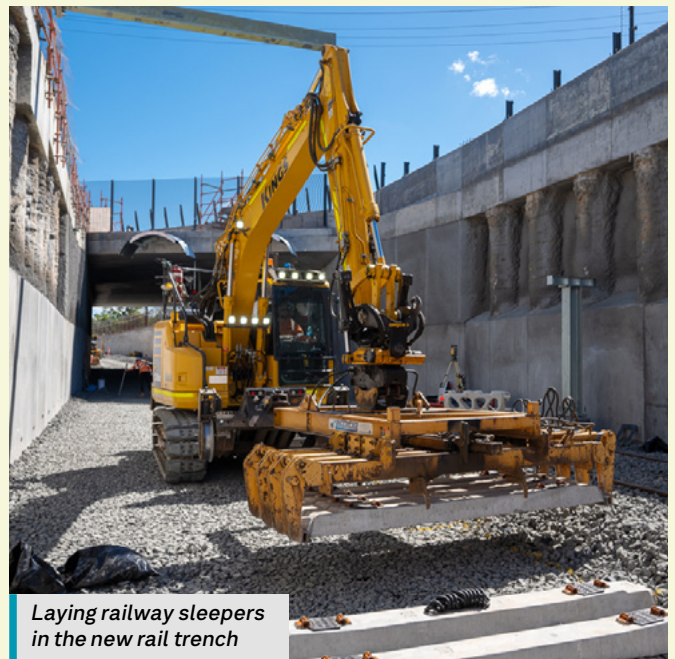
Construction work to build the new rail trench
