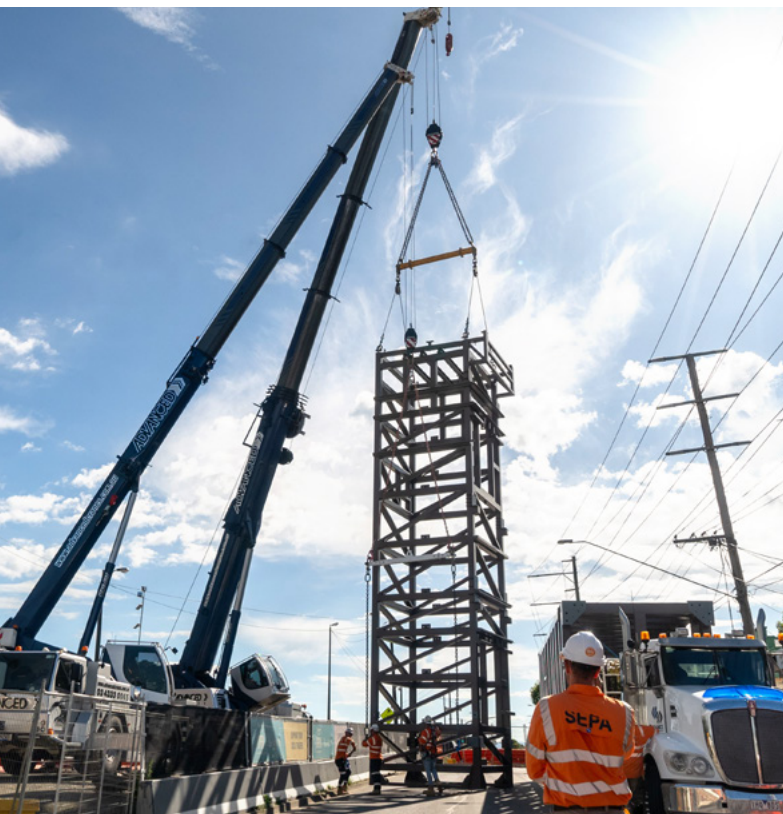
Crane lifting the lift shafts into place
