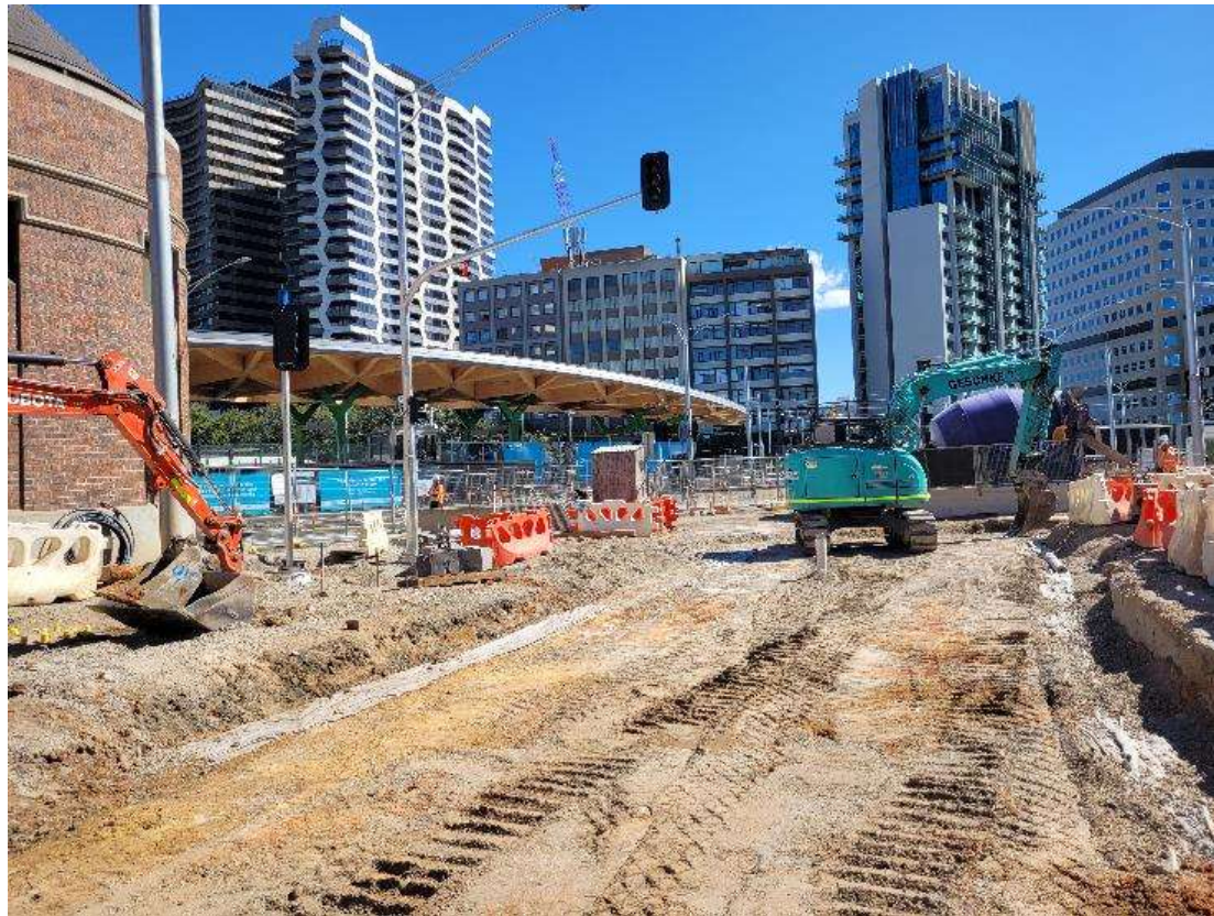
Domain Road rebuild
