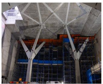
The ceiling for Town Hall Station's concourse at City Square is taking shape, with 8 columns standing up to 13.5 metres high, underneath one of the recently poured ground floor concrete slabs. This is where passengers entering from Collins Street will be able to touch on and make their way 30 metres below ground to the station platform.
