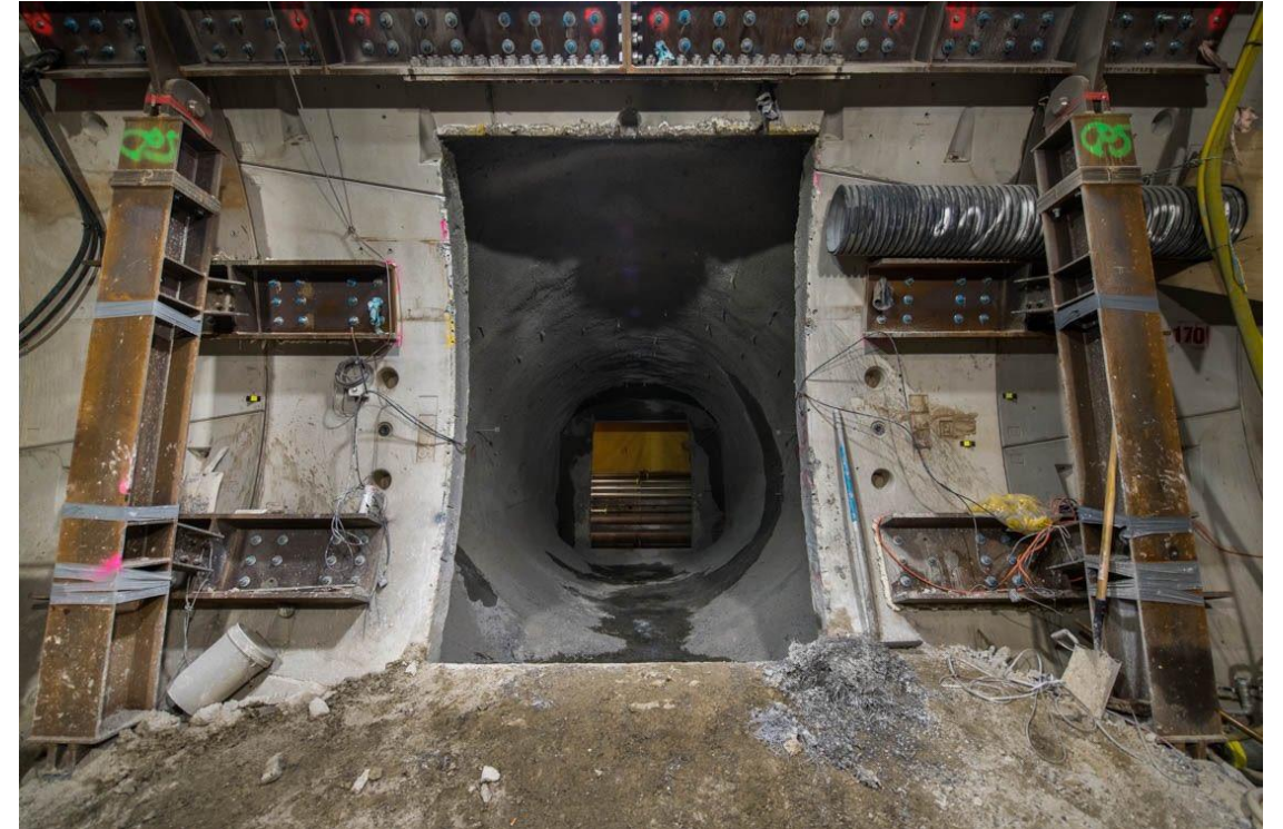
Cross passage construction as part of Metro Tunnel
