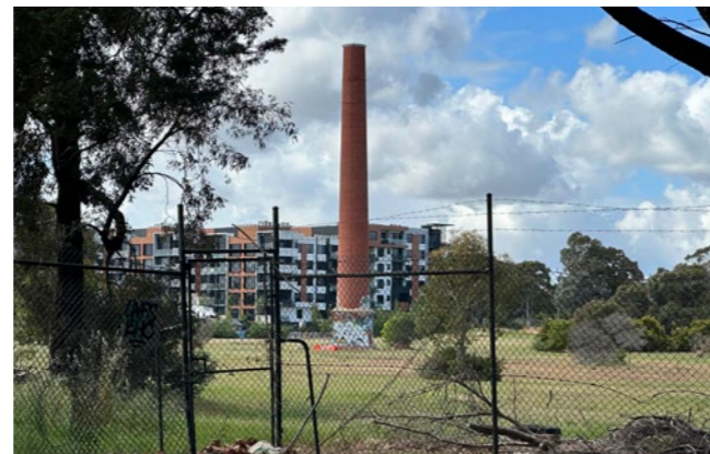
Figure 6.69: The existing boiler house chimney
