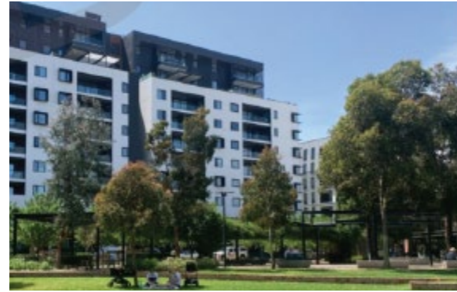
Figure 6.67: Example of the form of development envisaged for the Former Highett Gasworks Site
