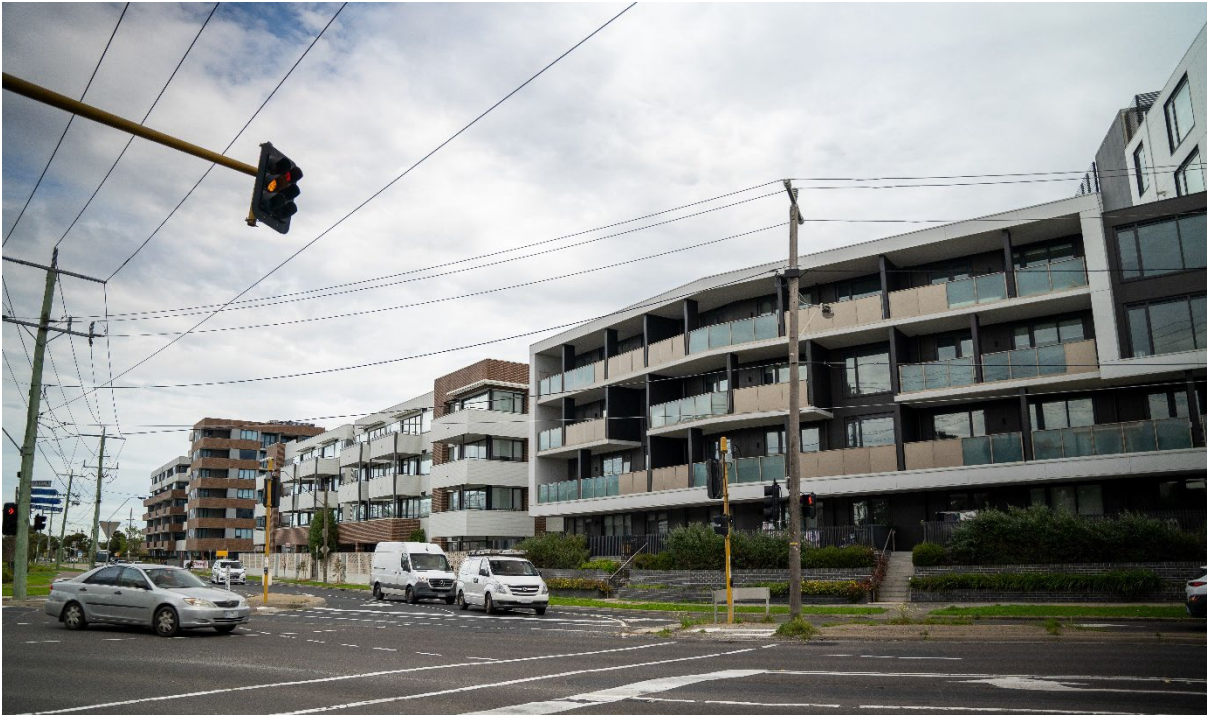
Existing apartment development in Clayton
