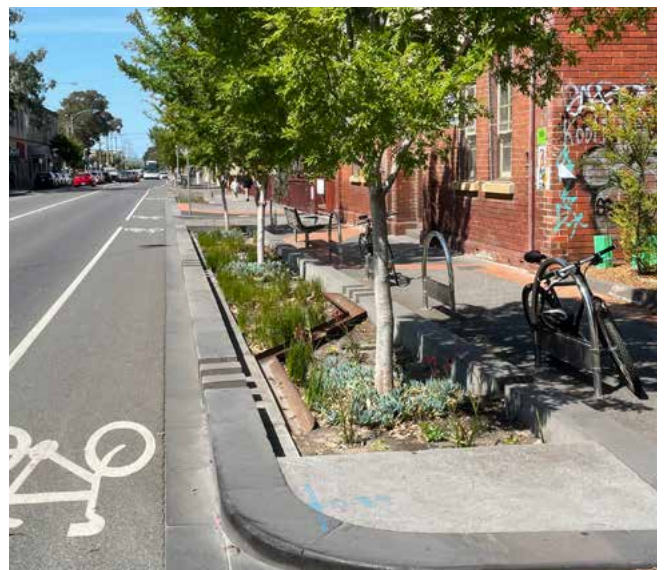
Example of Water Sensitive Urban Design on Dawson Street, Brunswick
