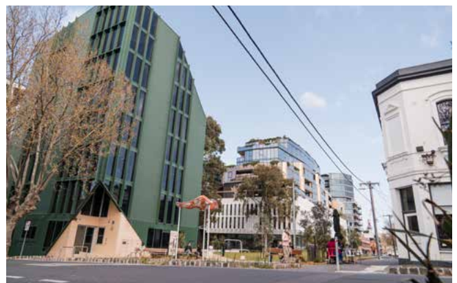
Example of a new office building and open space in Collingwood
