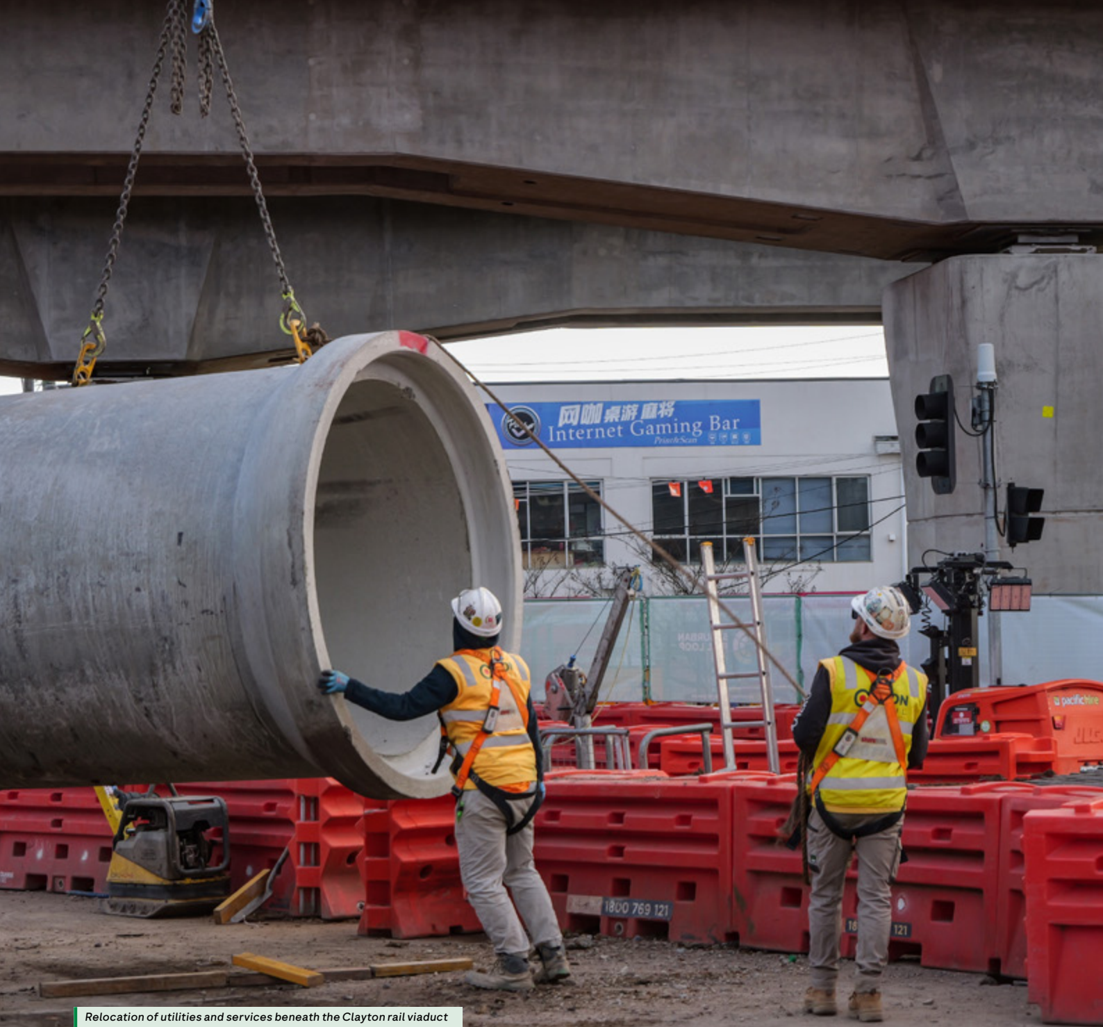
Relocation of utilities and services beneath the Clayton rail viaduct
