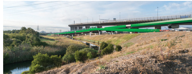
Hyde Street citybound exit ramp and walking and cycling path
