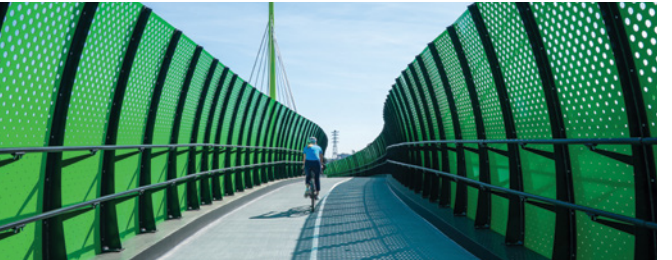
Footscray Road walking and cycling bridge
