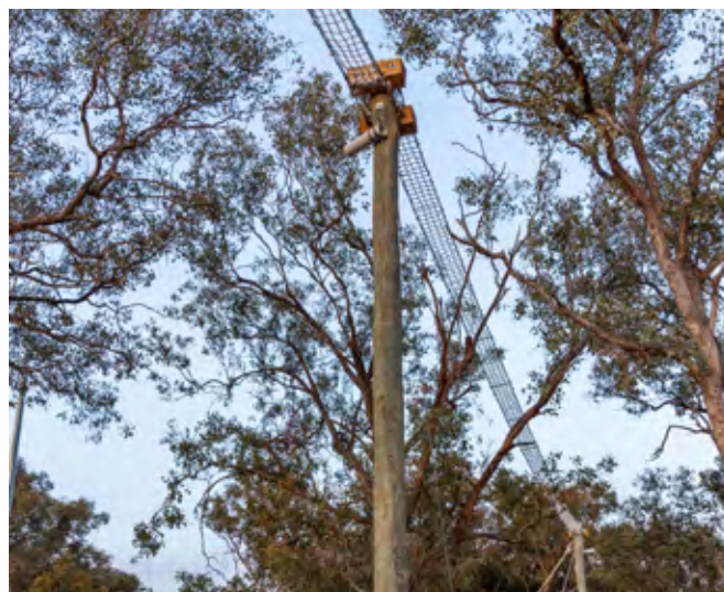
Photo 12 Canopy bridge for possums and gliders (Yan Yean Road; Source: VIDA Roads)
