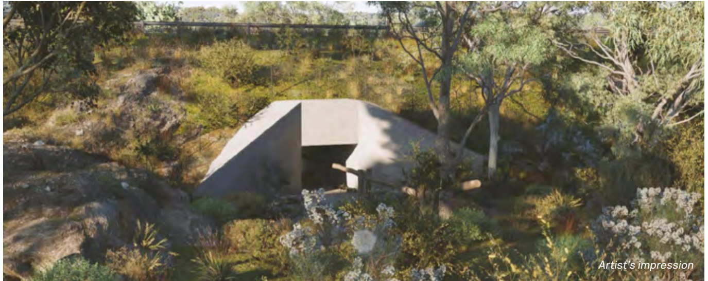
Figure 10 Virtual renders of large terrestrial culvert with lightwell and elevated wooden rail for arboreal fauna
