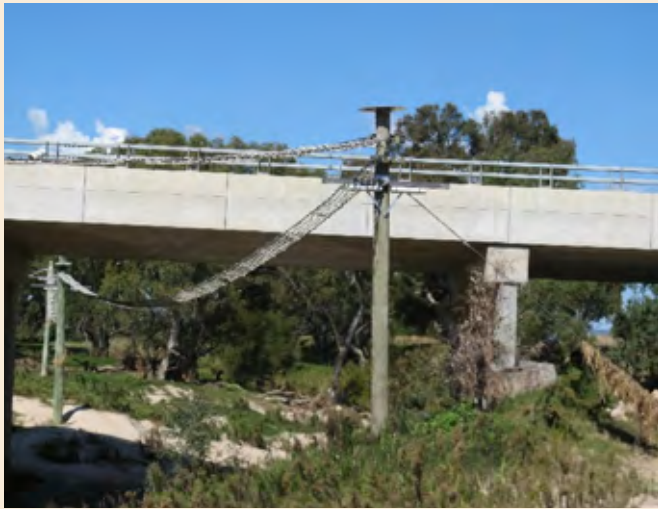
Photo 74 Canopy bridge under road bridge, Slaty Creek, Calder Freeway (Source: VicRoads)
