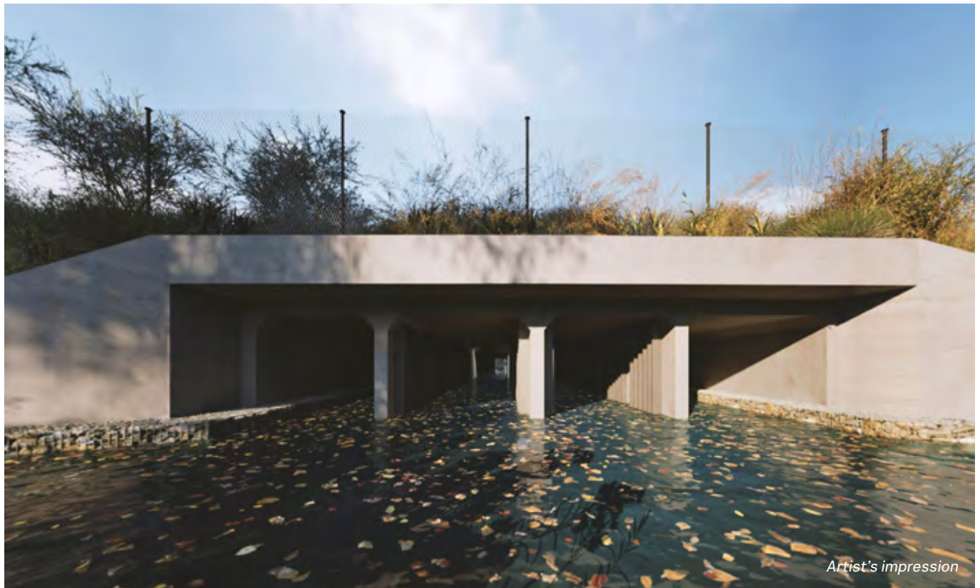
Figure 12 Virtual render of a multi-cell aquatic culvert concept design with baffles, light wells, and terrestrial ledge
