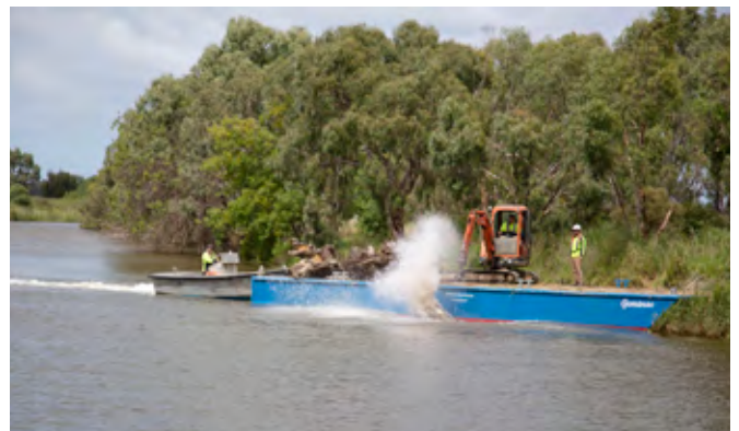
Photo 123 Tree root balls from Yan Yean Road – Stage 1 Upgrade being installed in Barwon River to create fish habitat (Source: Austin O'Malley, VIDA Roads)
