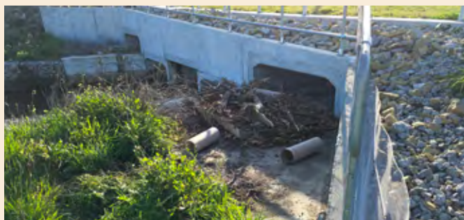
Photo 48 Drainage and ponding reduce culvert effectiveness; pipe culverts aren't ideal for fauna movement. (Source: Rodney van der Ree, WSP)
