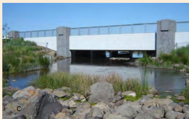
Photo 42 Sub-optimal Growling Grass Frog culvert, showing a lack of sufficient height/airspace and no dry passage options (Source: Jake Urlus, Tactecol)
