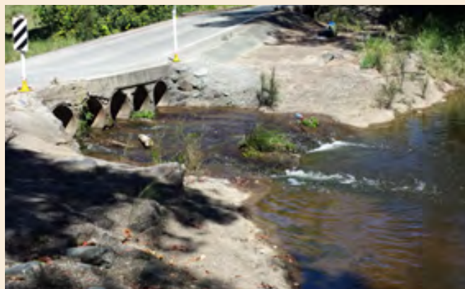
Photo 40 Integrating light wells into culverts facilitates fish passage – Fish Point fishway overpass on the Little Murray River (Source: Frank Amtstatter, Arthur Rylah Institute)
