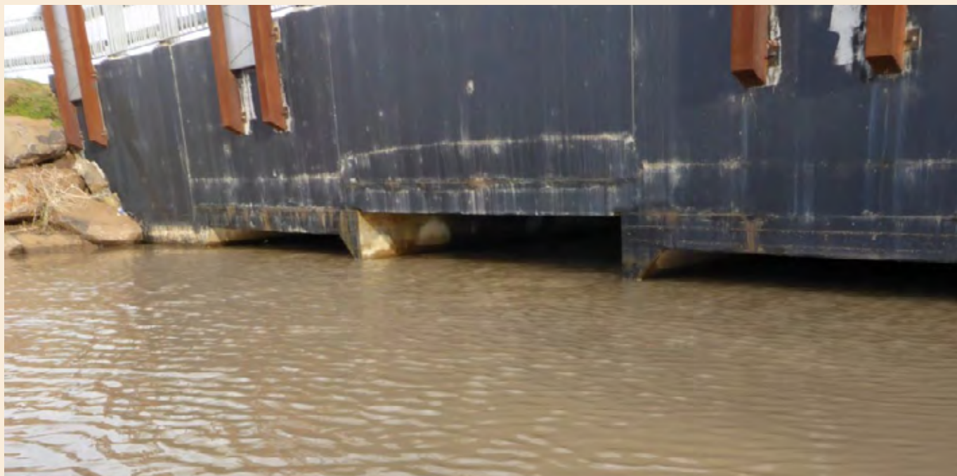
Photo 42 Sub-optimal Growling Grass Frog culvert, showing a lack of sufficient height/airspace and no dry passage options (Source: Jake Urlus, Tactecol)
