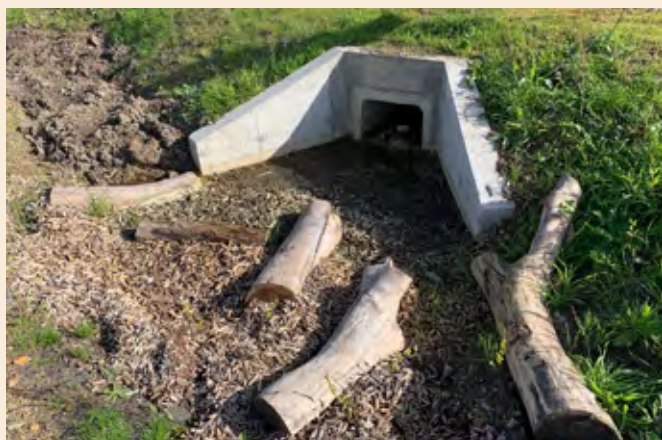
Photo 31 Small terrestrial culvert for bandicoots (Western Port Highway; Source: Austin O'Malley, VIDA Roads)
