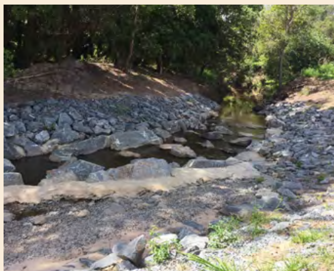
Photo 58 Fishway, Slacks Creek, QLD (Source: Craig Chargulaf, ARUP)
