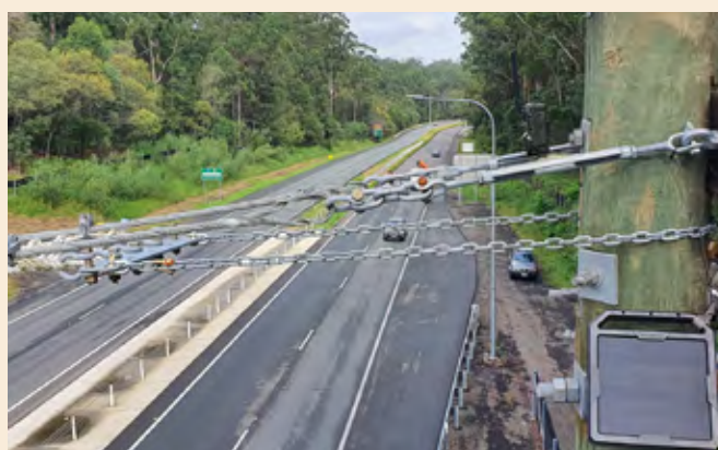
Photo 70 Example of poor design – The rope ladder is connected to the pole via 1 m of steel cable. The ladder should connect directly to the pole to improve ease of access (Source: Rodney van der Ree, WSP)
