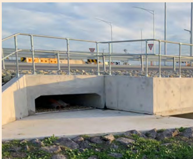
Photo 15 Small pre-cast wildlife culvert under a narrow sealed access road in the Royal Botanic Gardens Cranbourne (Source: Royal Botanic Gardens Cranbourne)
