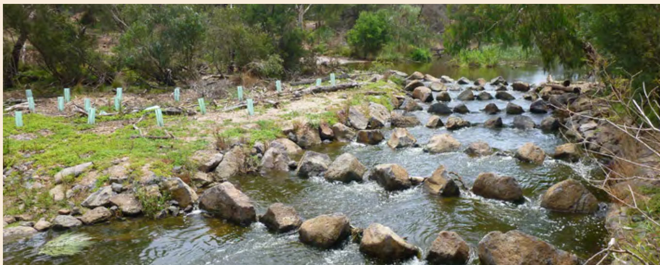
Photo 55 Fishway, Coburg Lake, Victoria (Source: Clio Gates Foale, VIDA Roads)
