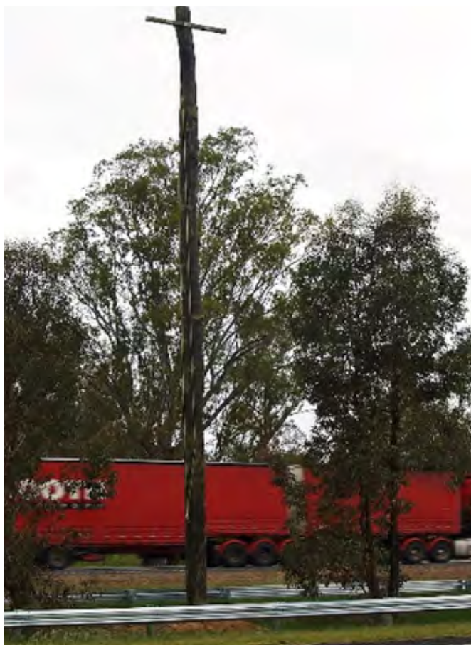
Photo 80 Glider pole installed in centre median of Hume Freeway, Victoria. Cross-arm should be perpendicular to the road and point towards the opposite side of the road (Source: Rodney van der Ree, WSP)
