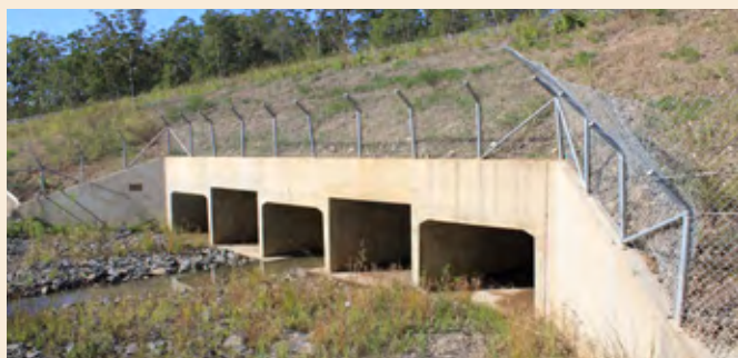
Photo 52 Example of strategies that provide dry passage if the culvert contains standing or flowing water (Source: Rodney van der Ree, WSP)
