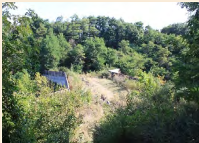
Photo 61 Land bridge in France showing noise and light screens and different habitats for different species, i.e., a row of tree stumps, short grass down the centre and shrubs on both sides (Source: Rodney van der Ree, WSP)
