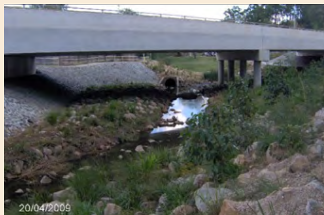
Photo 25 Example of a sub-optimal bridge underpass — minimal terrestrial wildlife zone and over-use of large rocks for erosion control (Source: Rodney van der Ree, WSP)
