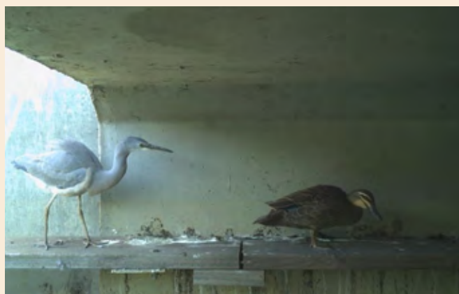
Photo 38 Example of poor culvert design for aquatic fauna (Source: Andrea McPherson, ARUP)
