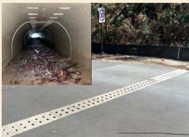
Photo 15 Small pre-cast wildlife culvert under a narrow sealed access road in the Royal Botanic Gardens Cranbourne (Source: Royal Botanic Gardens Cranbourne)
