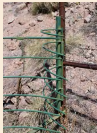
Photo 89 Example of one-way gate from the USA (left) and jump out from the Pacific Highway NSW (right) (Source: Rodney van der Ree, WSP)
