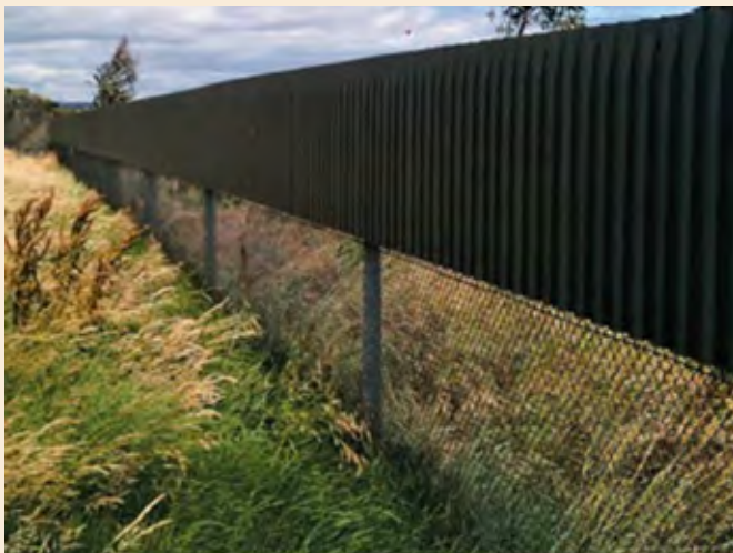
Photo 86 Temporary fencing for Growling Grass Frog (Source: Aidan Cresser, VIDA Roads)
