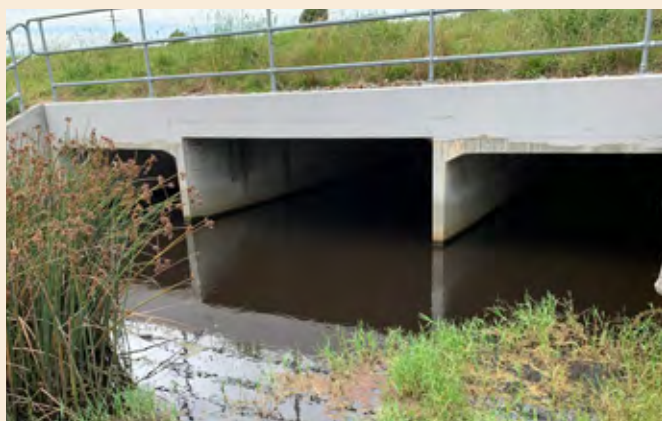
Photo 37 Aquatic culverts, Princes Highway, Victoria (Source: Austin O'Malley, VIDA Roads)
