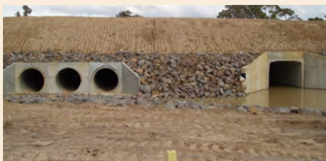
Photo 51 Slab-link multi-use culverts as per photo 50 (Source: Rodney van der Ree, WSP)
