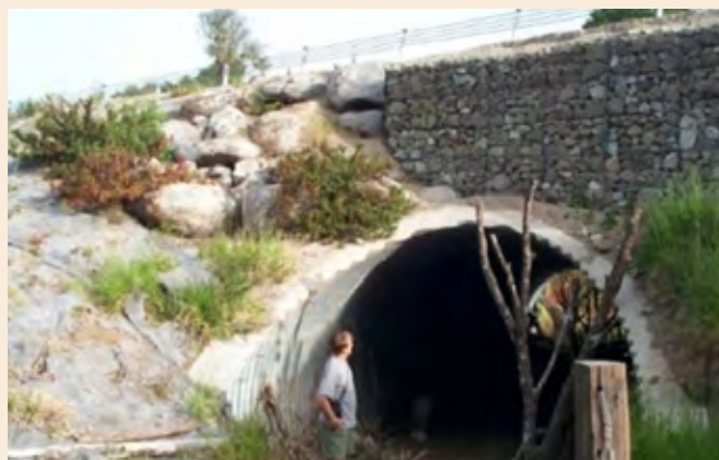
Photo 30 Microclimate vents within the centre median of the Princes Highway, Victoria (Source: Austin O'Malley, VIDA Roads)
