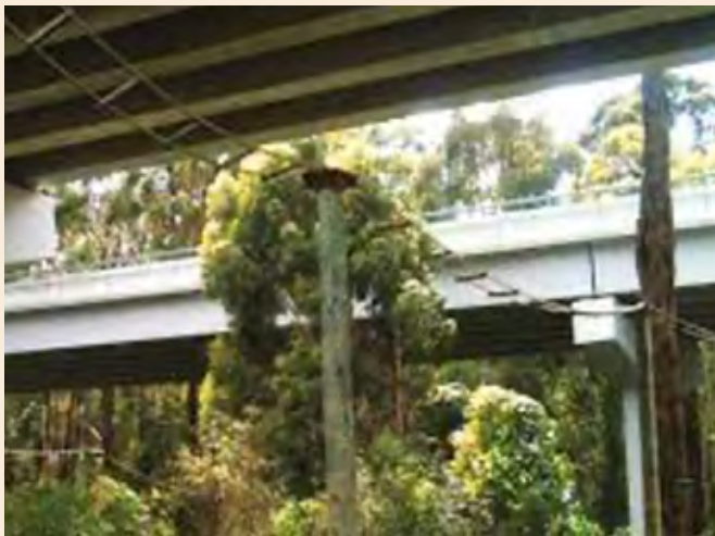
Photo 76 Canopy bridge under Echuca-Moama Bridge (Source: VIDA Roads)
