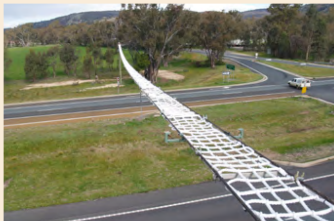
Photo 66 Canopy bridge across the Hume Freeway, central Victoria, showing the flat rope ladder attached to two steel cables (Source: Rodney van der Ree, WSP)
