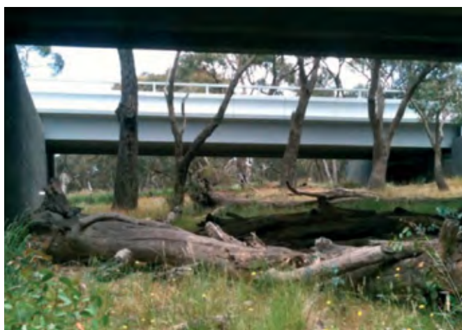
Photo 103 Example fauna furniture and natural shelters – large logs laid on the ground beneath the Calder Freeway (Source: VicRoads)
