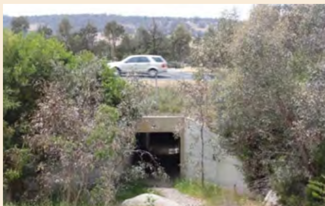
Photo 29 The first arch underpass for birds, located on the Hume Highway at Woomargama NSW (Source: Rodney van der Ree, WSP)
