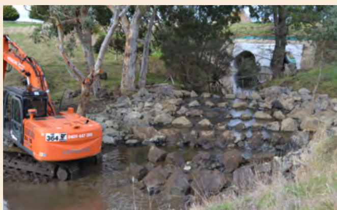
Photo 39 Existing or new pipe culverts can be drowned-out by the addition of a fishway downstream – Muddy Creek, southwest Vic (Source: Ivor Stuart, Arthur Rylah Institute)
