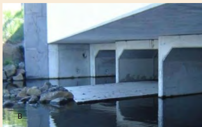
Figure 13 Successful culvert design for the threatened Growling Grass Frog (DELWP 2017); originally reproduced from Koehler and Gilmore (2014) and all images Daniel Gilmore, Biosis Pty Ltd.
