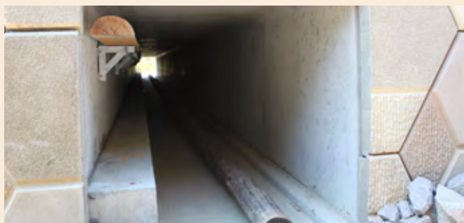
Photo 52 Example of strategies that provide dry passage if the culvert contains standing or flowing water (Source: Rodney van der Ree, WSP)
