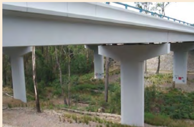
Photo 23 Example of a well-designed bridge underpass — open with natural substrate and continuous vegetation (Source: Rodney van der Ree, WSP)
