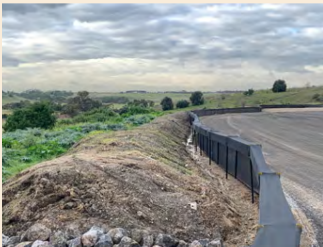
Photo 88 Escape ramp for Koalas on W2B Pacific Hwy Upgrade, NSW (Source: Rodney van der Ree, WSP)
