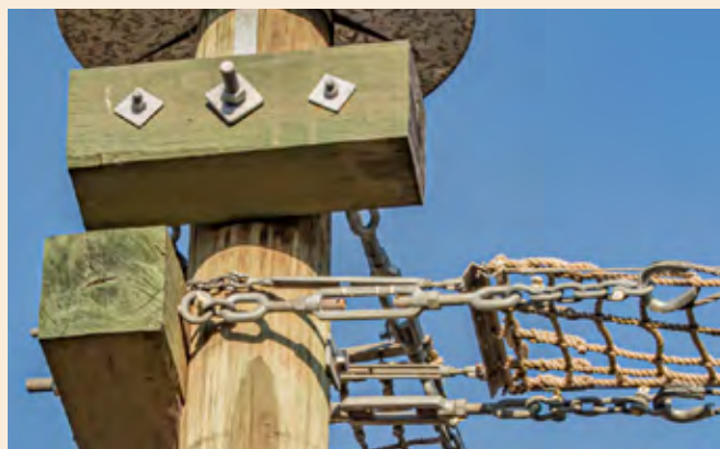
Photo 68 Close up of connection of rope ladder to the supporting pole. The rope ladder should extend all the way to the pole to improve ease of access for possums, gliders and other arboreal animals (Source: Rodney van der Ree, WSP)
