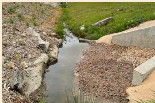
Photo 32 Drainage requires consideration to ensure terrestrial fauna culverts remain dry and free draining after flooding (Western Port Highway; Source: Austin O'Malley, VIDA Roads)
