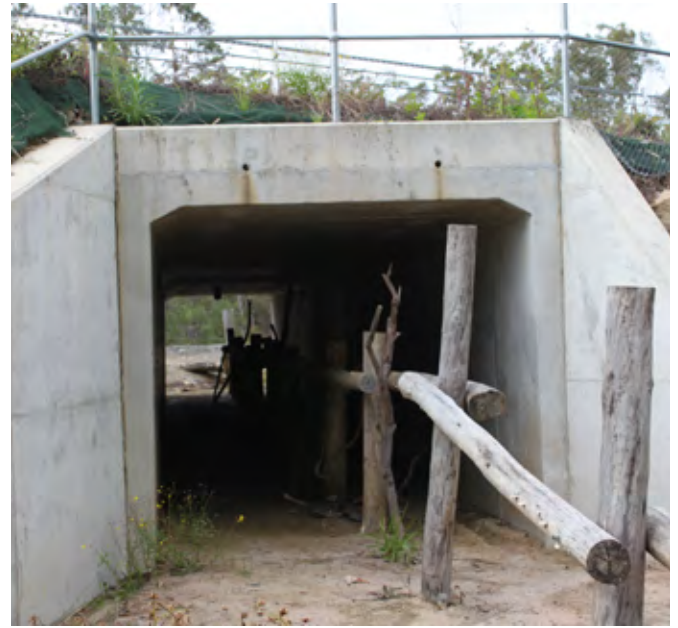
Photo 108 Bandicoot hide, Healesville-Koo Wee Rup Road Upgrade (Source: Austin O'Malley)
