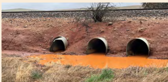
Photo 50 Slab-link multi-use culverts on the Pacific Highway NSW. Middle cell designed to take water year-round, outer cells remaining dry except during flood events (Source: Rodney van der Ree, WSP)
