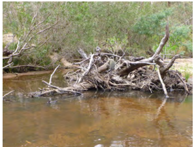
Photo 123 Tree root balls from Yan Yean Road – Stage 1 Upgrade being installed in Barwon River to create fish habitat (Source: Austin O'Malley, VIDA Roads)
