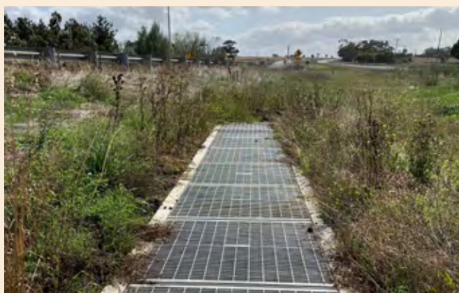
Photo 32 Drainage requires consideration to ensure terrestrial fauna culverts remain dry and free draining after flooding (Western Port Highway; Source: Austin O'Malley, VIDA Roads)
