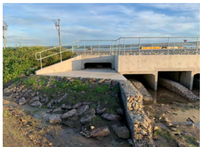
Photo 44 Multi-use culvert for terrestrial small mammals (left) and amphibian (right) passage (VIDA Roads Healesville-Koo Wee Rup Road Upgrade project (Source: Austin O'Malley, VIDA Roads)
