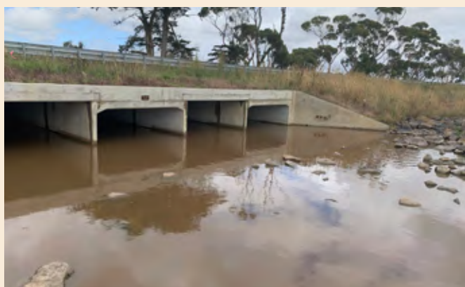
Photo 39 Existing or new pipe culverts can be drowned-out by the addition of a fishway downstream – Muddy Creek, southwest Vic (Source: Ivor Stuart, Arthur Rylah Institute)
