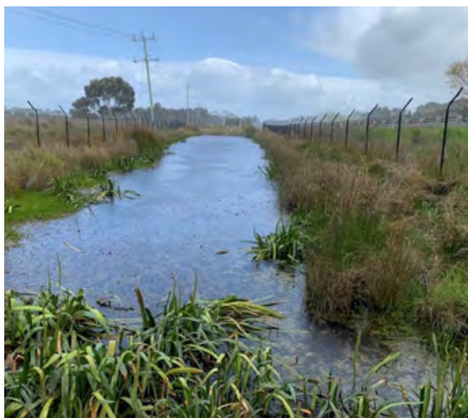
Photo 117 Constructed frog pond with emergent and floating vegetation (Princess Highway Duplication; Source: Austin O'Malley, VIDA Roads)
