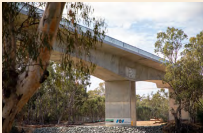
Photo 24 Example of a sub-optimal bridge underpass — lack of terrestrial wildlife zone and over-use of large rocks for erosion control (Source: Austin O'Malley, VIDA Roads)
