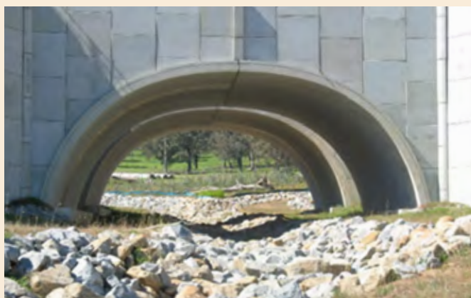
Photo 31 Small terrestrial culvert for bandicoots (Western Port Highway; Source: Austin O'Malley, VIDA Roads)
