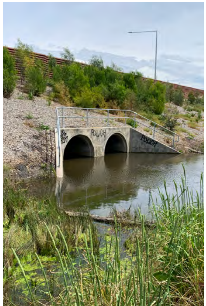
Photo 34 Aquatic culvert for incidental fish passage in low-flow contexts (Mordialloc Freeway; Source: Austin O'Malley, VIDA Roads)
