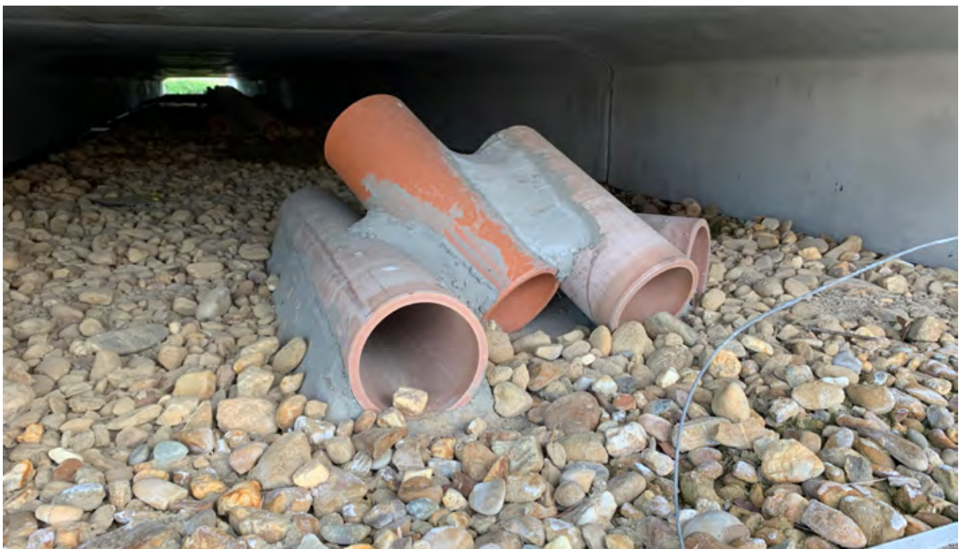
Photo 106 Terracotta pipe pile shelter and natural floor treatment (Healesville-Koo Wee Rup Road Upgrade; Source: Austin O'Malley, VIDA Roads)
