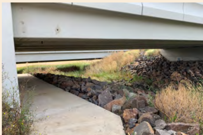
Photo 24 Example of a sub-optimal bridge underpass — lack of terrestrial wildlife zone and over-use of large rocks for erosion control (Source: Austin O'Malley, VIDA Roads)
