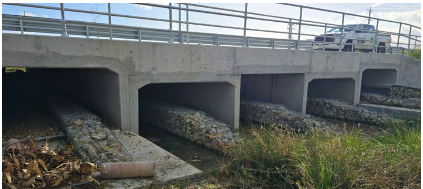
Photo 45 A multi-use type crossing design for threatened Southern Brown Bandicoots (small marsupial) and Growling Grass Frog (amphibian) on the VIDA Roads Healesville–Koo Wee Rup Upgrade project. Note gabion basket ramps and terrestrial ledge on outside culverts. (Source: Austin O'Malley, VIDA Roads)
