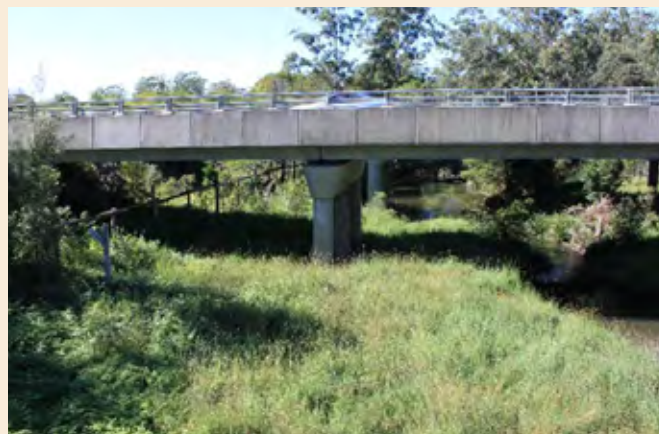
Photo 25 Example of a sub-optimal bridge underpass — minimal terrestrial wildlife zone and over-use of large rocks for erosion control (Source: Rodney van der Ree, WSP)
