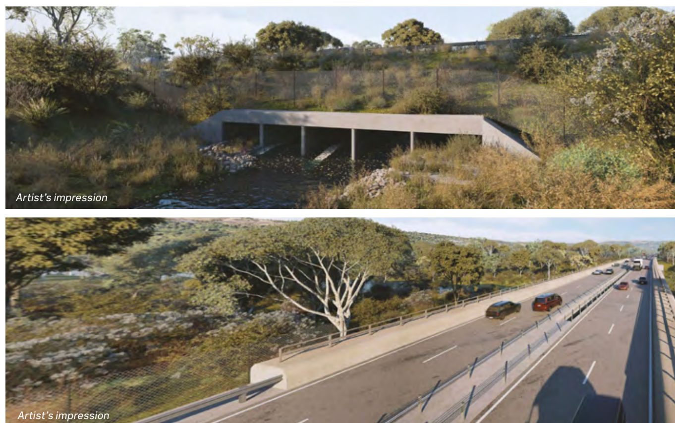
Figure 30 Example conceptual render of wildlife exclusion fencing integrated into a culvert crossing (top) and wildlife bridge underpass (bottom)
