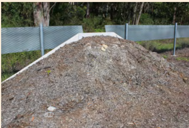
Photo 88 Escape ramp for Koalas on W2B Pacific Hwy Upgrade, NSW (Source: Rodney van der Ree, WSP)
