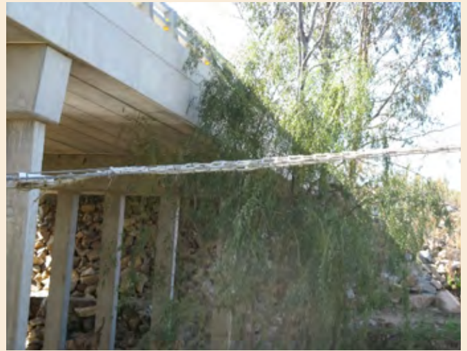
Photo 75 Canopy bridge under road bridge, Slaty Creek, Calder Freeway (Source: VicRoads)
