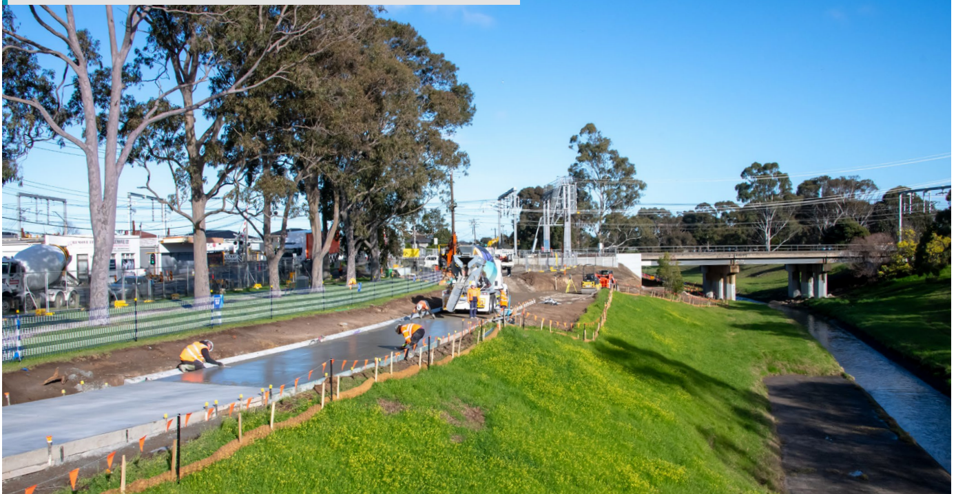
Construction of the new walking and cycling path along Webster Street
