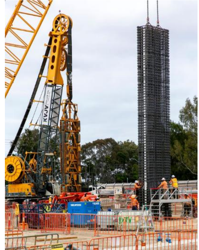
Steel cage for D-wall lowered into place at Heatherton.
