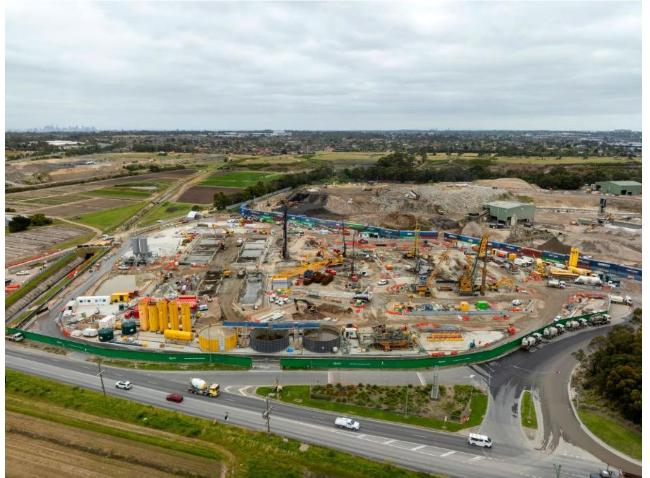
Clarinda worksite (December 2025)
