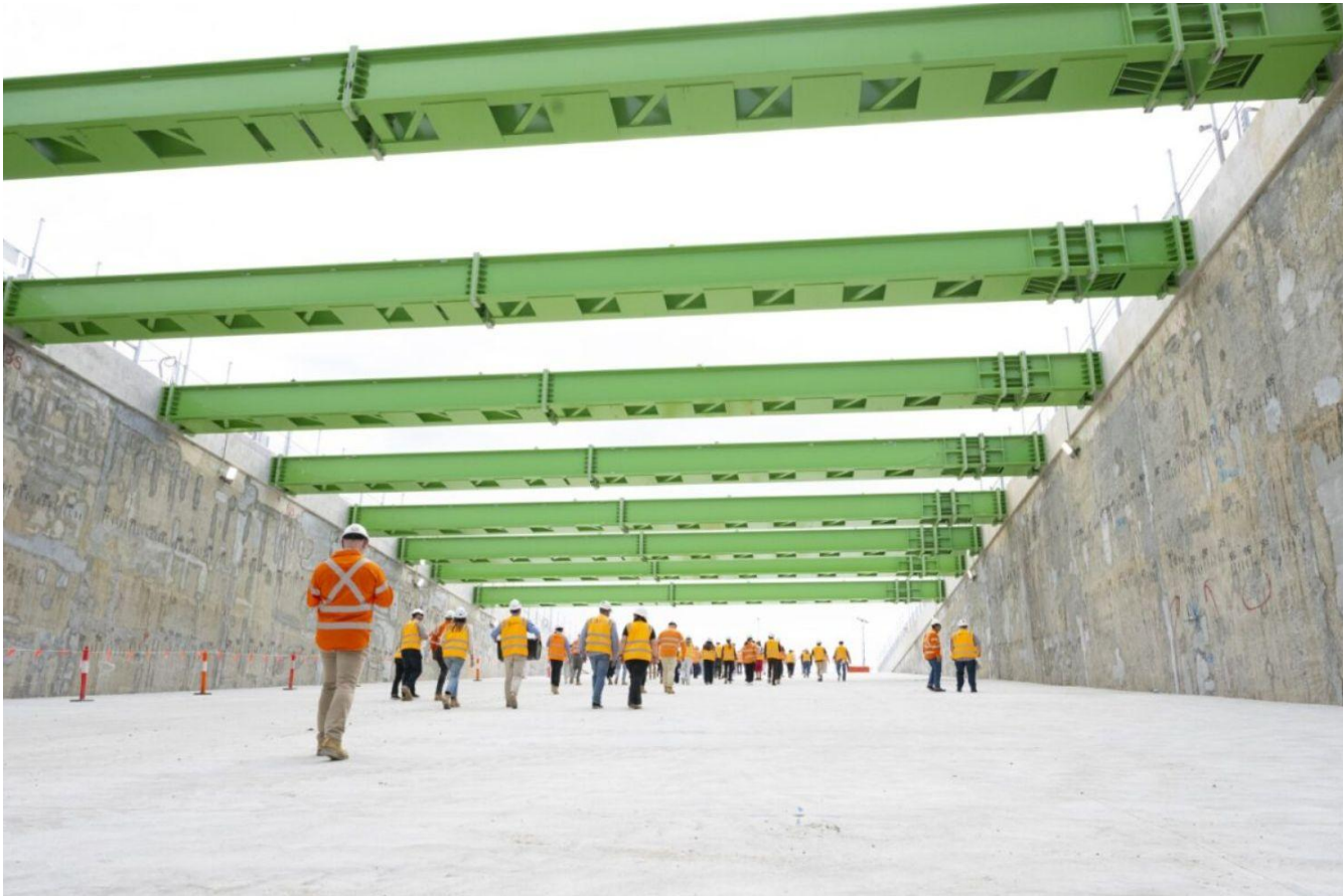
Heatherton eastern tunnel entrance – site handed over to Suburban Connect early 2026
