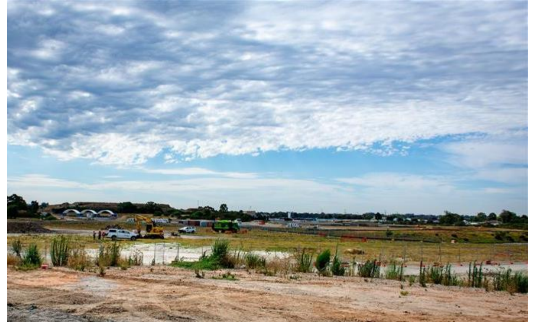
Site investigations at train stabling facility
