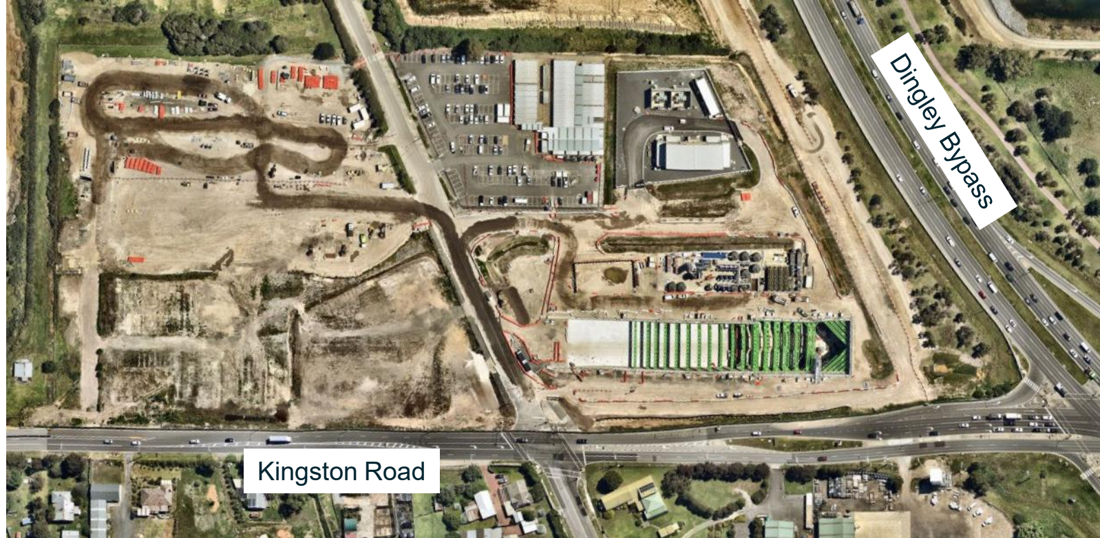
Eastern tunnel entrance site (December 2025)
