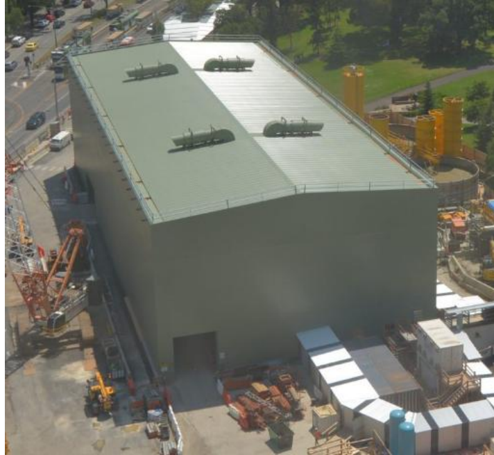
Example: Metro Tunnel Acoustic Shed at ANZAC Station.
