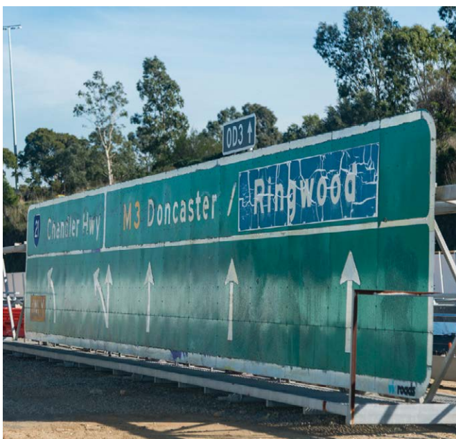
Overhead signage removal - Eastern Freeway near Hoddle Street
