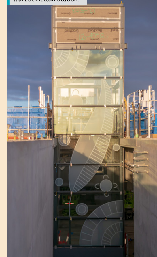
Co-design elements on a lift at Melton Station.
